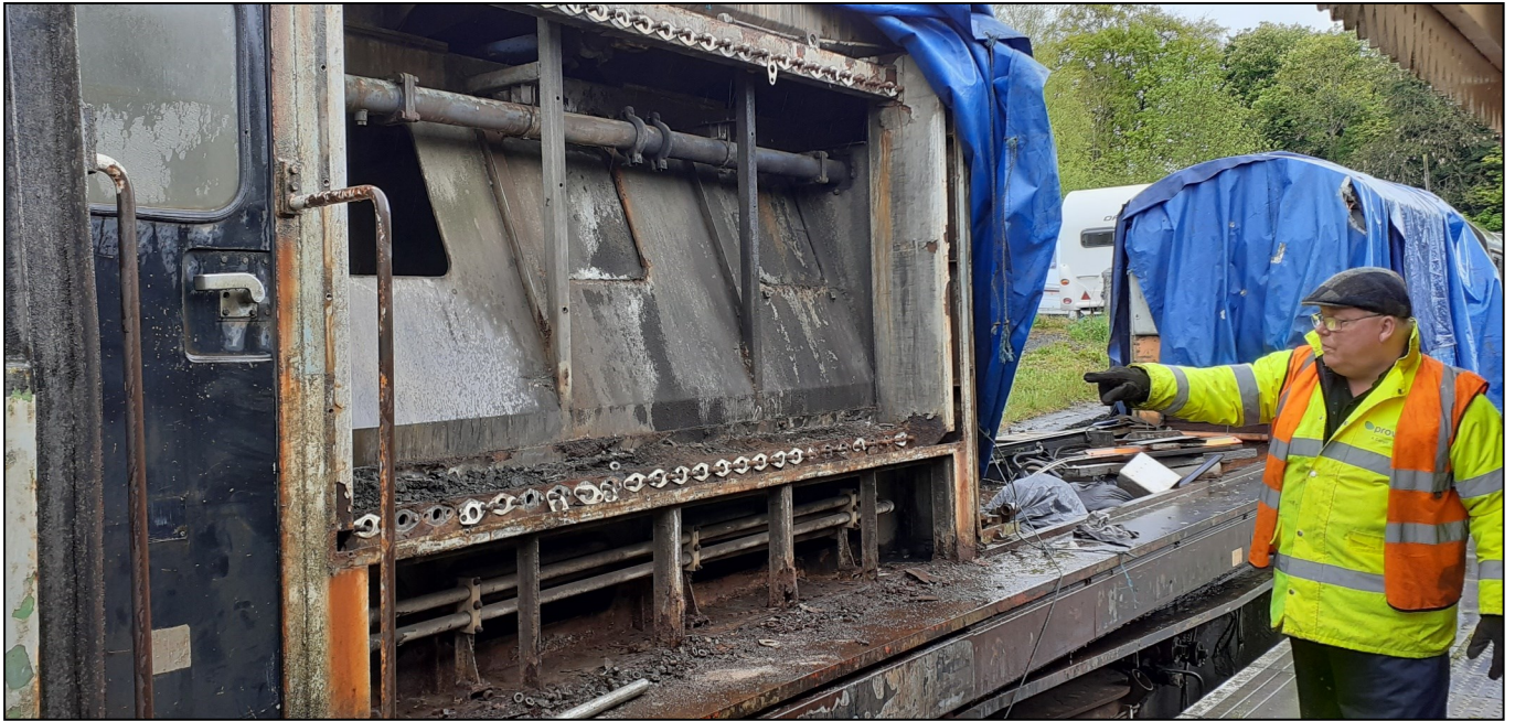
Above: Tony explaining how he and Phil managed to get the last, and most stubborn elements out of the radiator. Below: the effect of 20 years of wet coal dust on steel nuts.
