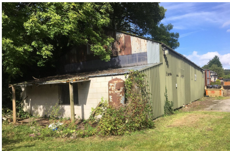
The storage area on the back of the workshop
