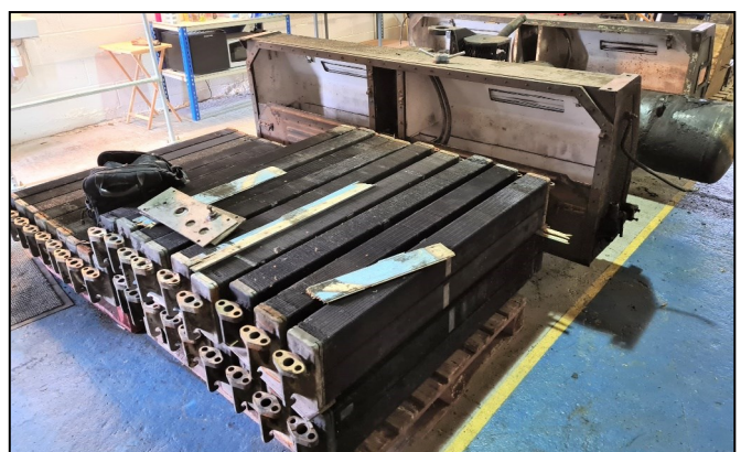
Right: Radiator elements and one of the battery boxes removed from 58022.
