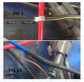
Slide the heat the shrink tube over the join and reduce. See **FIG 5A**
