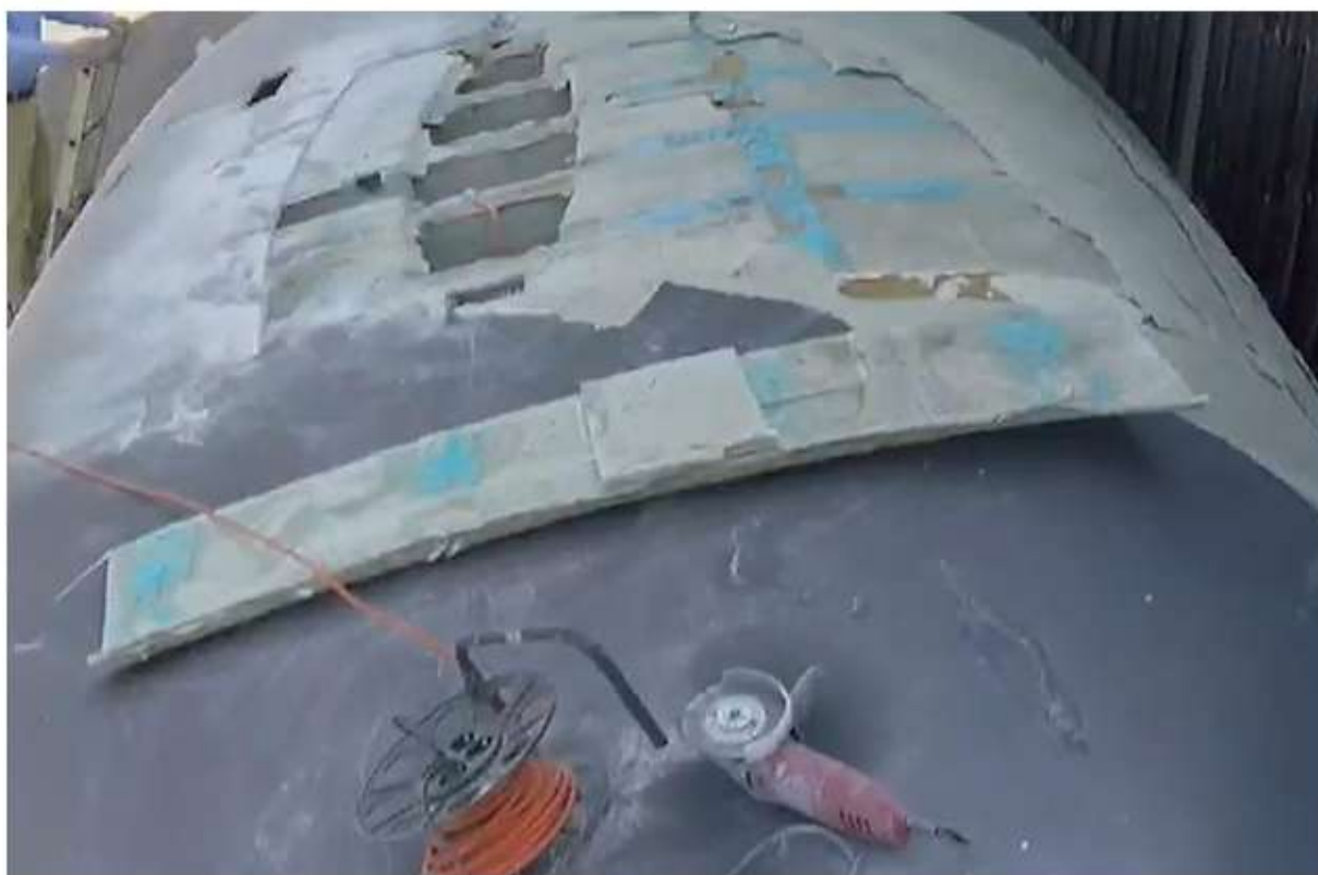
Photograph 7. Strip of sheathing cut out by the yacht owner (source: yacht owner)
