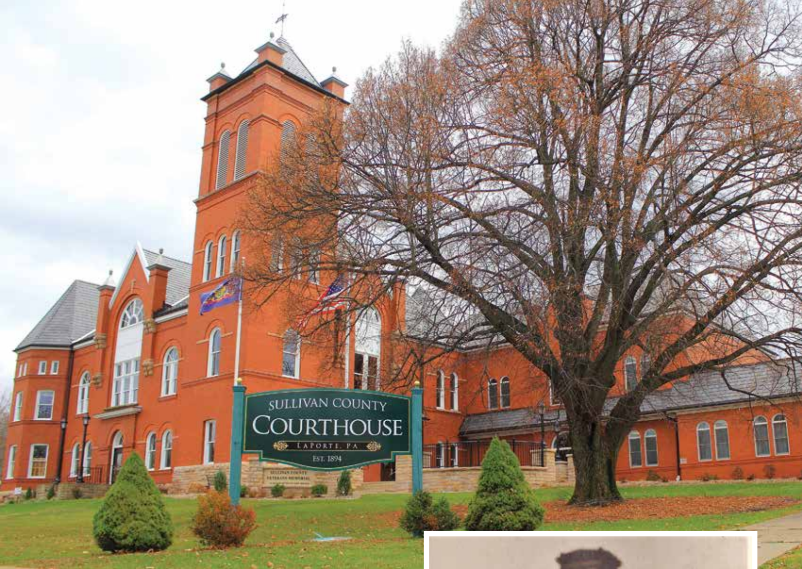
The current Sullivan County Courthouse
