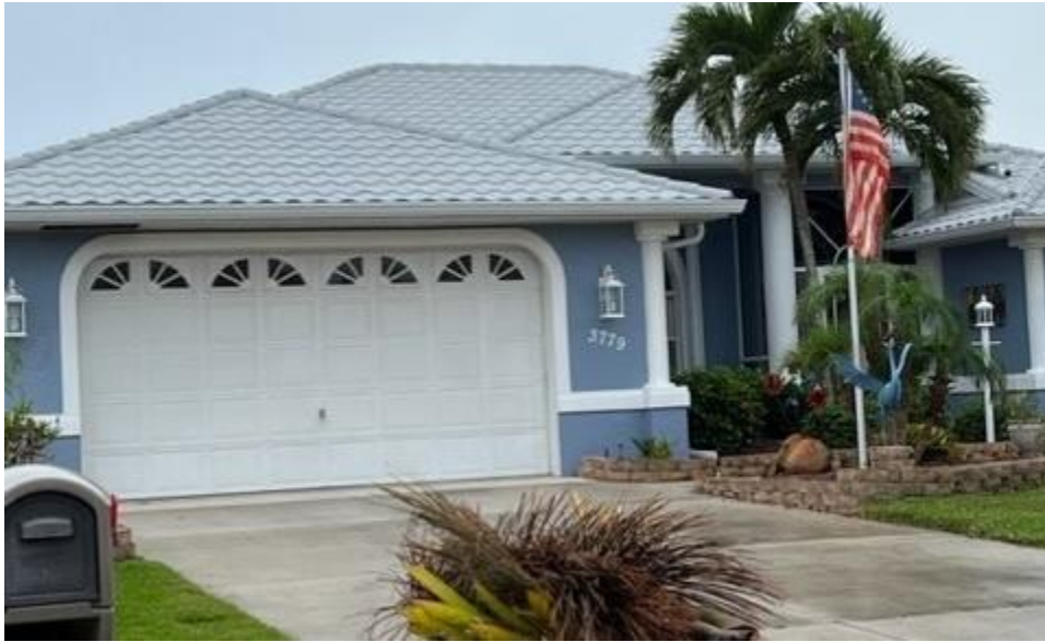
Example of BSI metal tile roof
