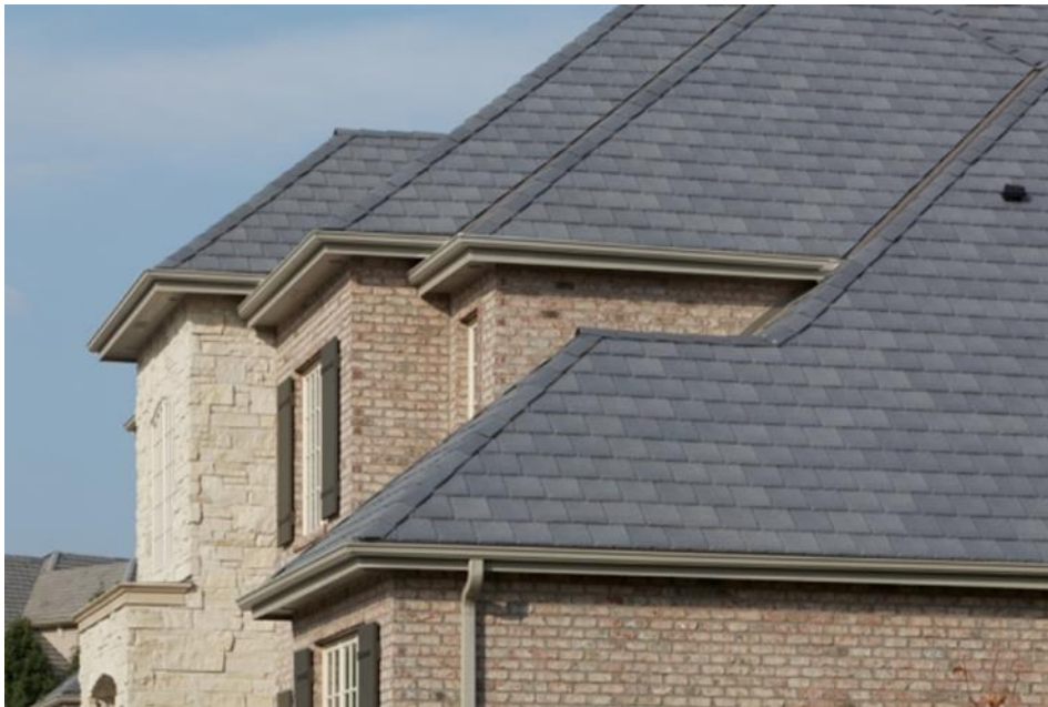
Example of Composite Synthetic Tile
