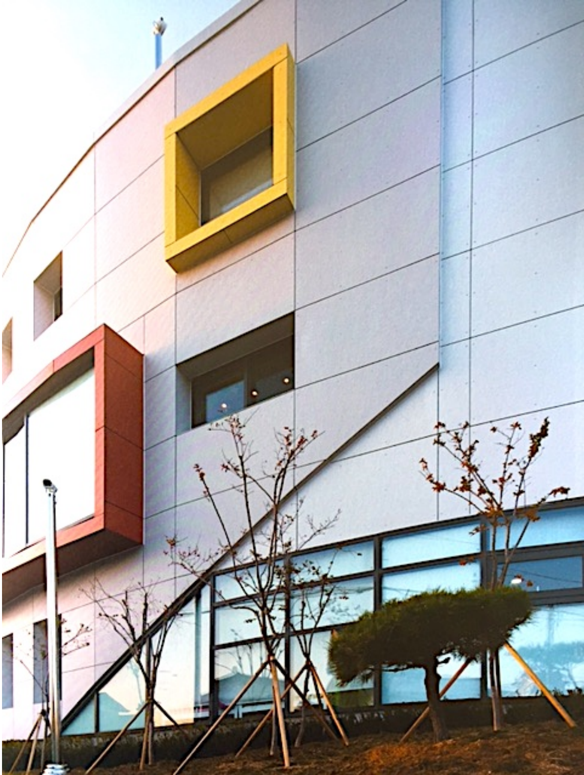
Figure 21: Example of wall cladding on building façade.
