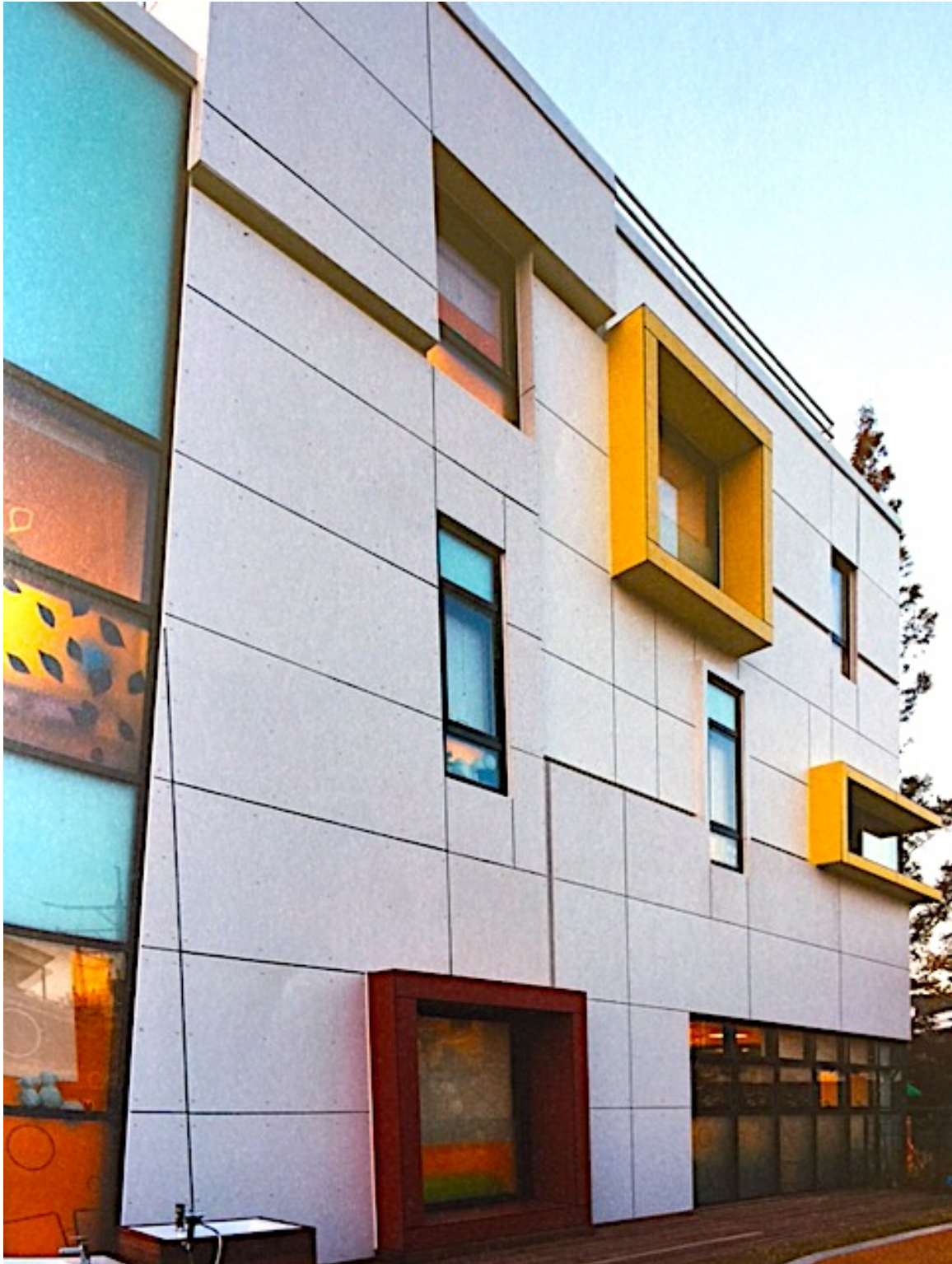
Figure 20: Example of wall cladding on building façade.
