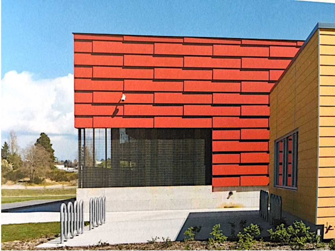
Figure 22: Example of wall cladding on building façade.
