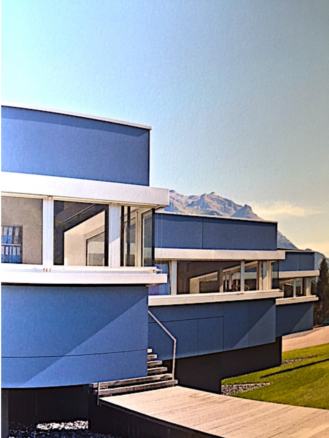
Figure 24: Example of wall cladding on building façade.
