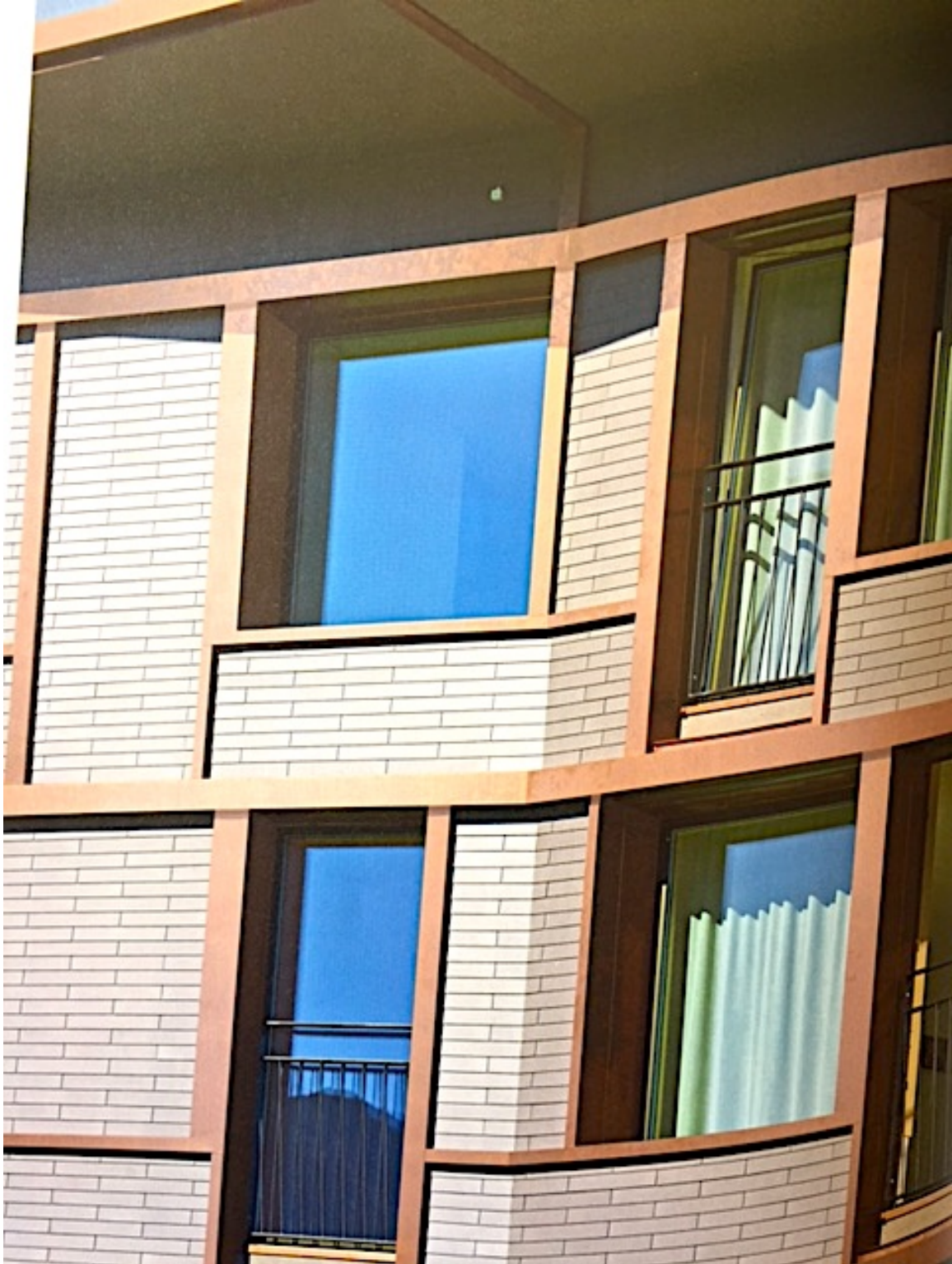
Figure 23: Example of wall cladding on building façade.
