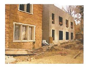
Concrete block and brick masonry
