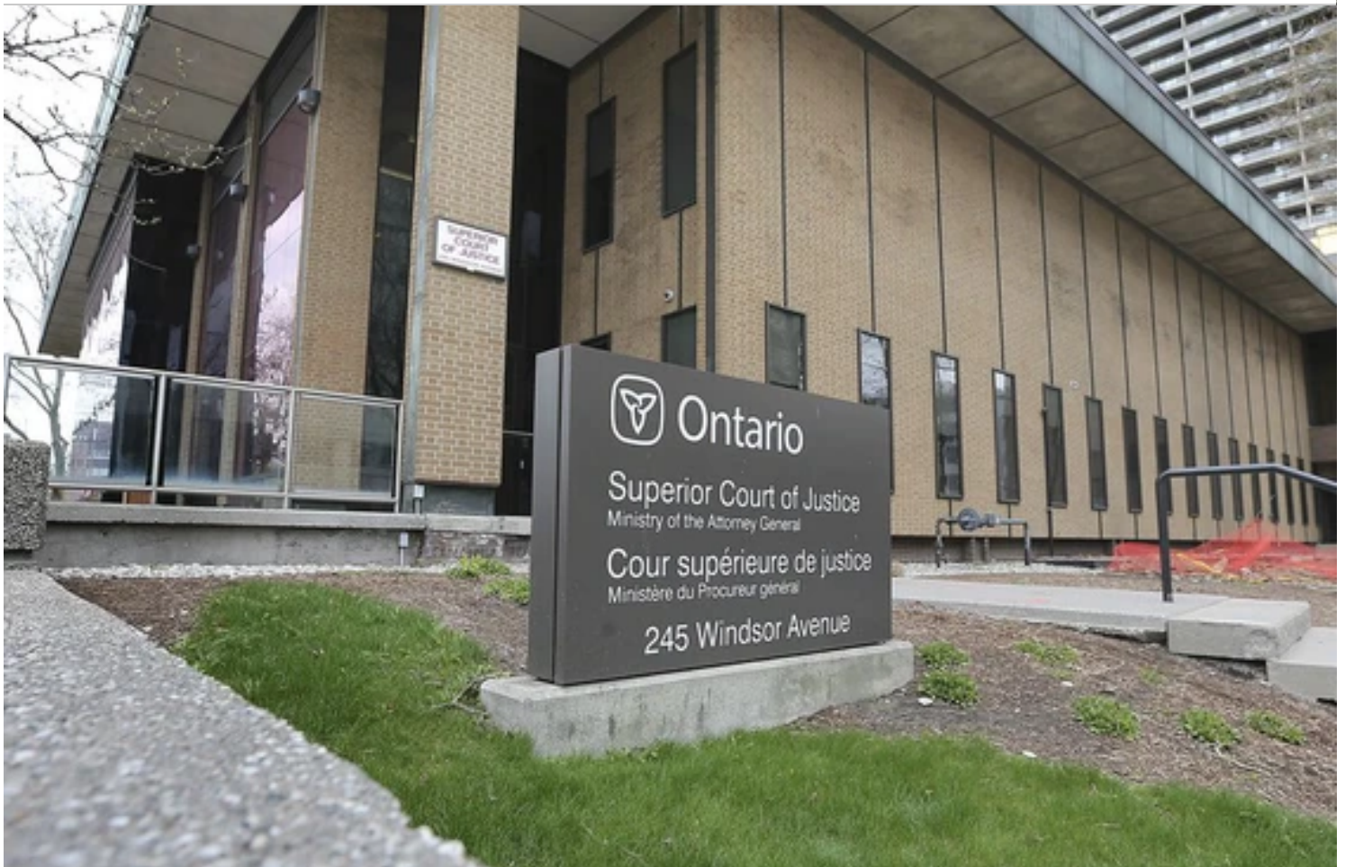
The exterior of the Superior Court of Justice in Windsor is shown on Thursday, April 22, 2021. PHOTO BY DAN JANISSE /Windsor Star
