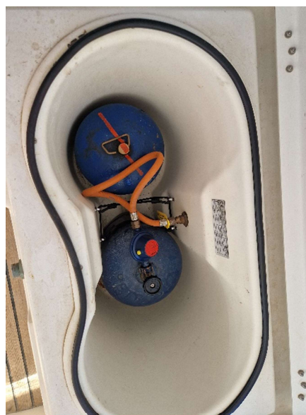
Gas installation with safety device for oven
