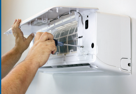
Back out electrical panel screws
