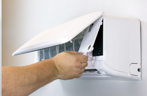
Remove electrical access panels (2)
