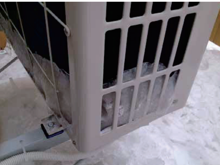
Without the right technology, condensate freezes to the bottom of the unit and reduces its efficiency and heating output.
