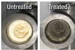
Water heater outlet
