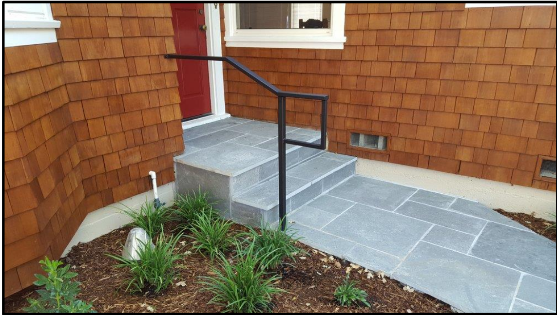
Pathway and front stoop: Bluestone over concrete San Anselmo, CA
