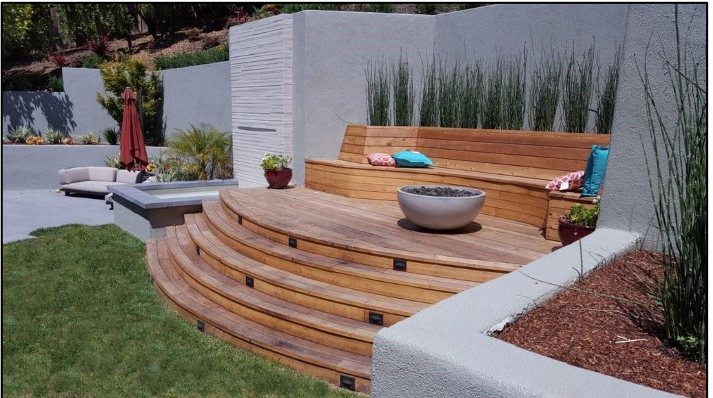
Custom curved redwood deck with S-Turn seat bench, integrated planter box seatback, installation of natural gas fire bowl. Custom programmable stair lighting. Custom water feature. Mill Valley, CA
