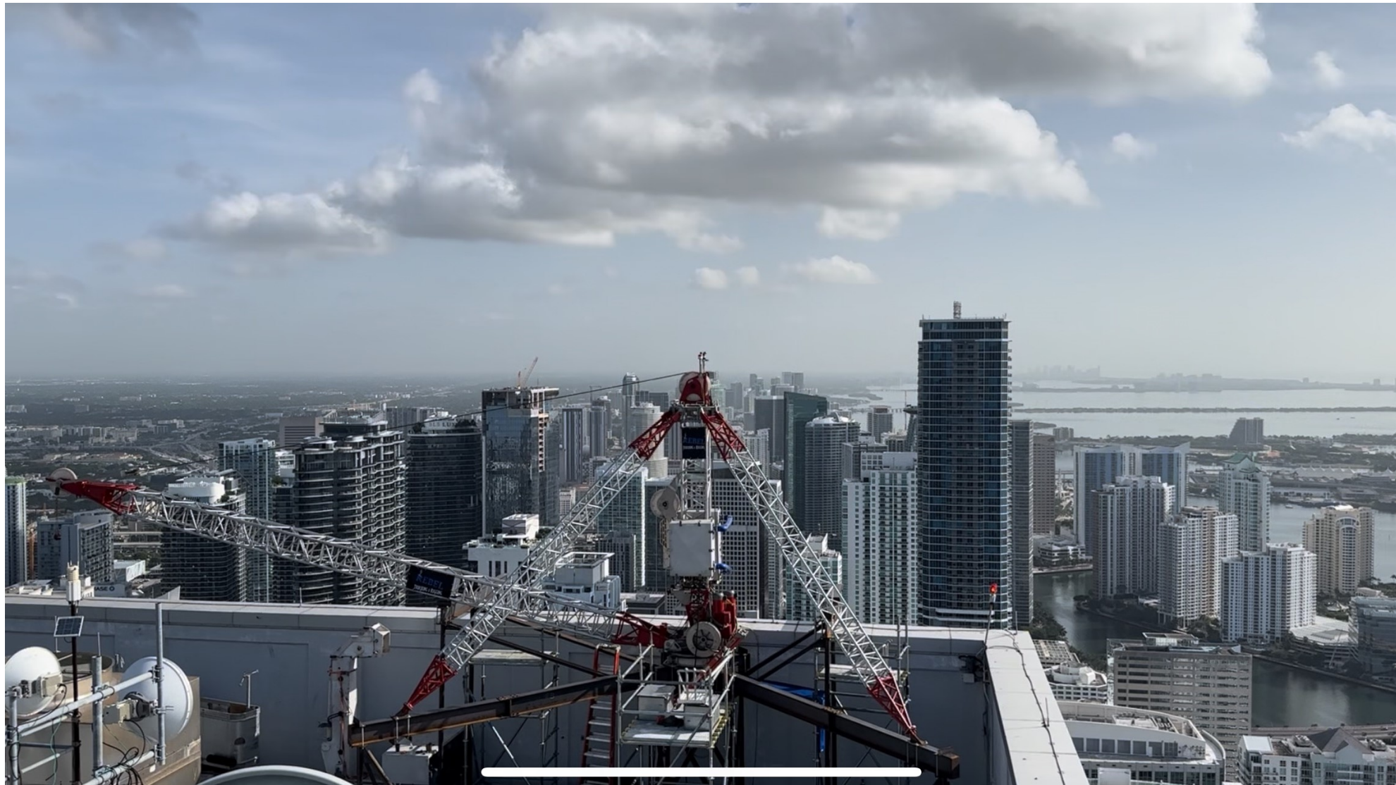
LSC on support beams 820' above sidewalk
