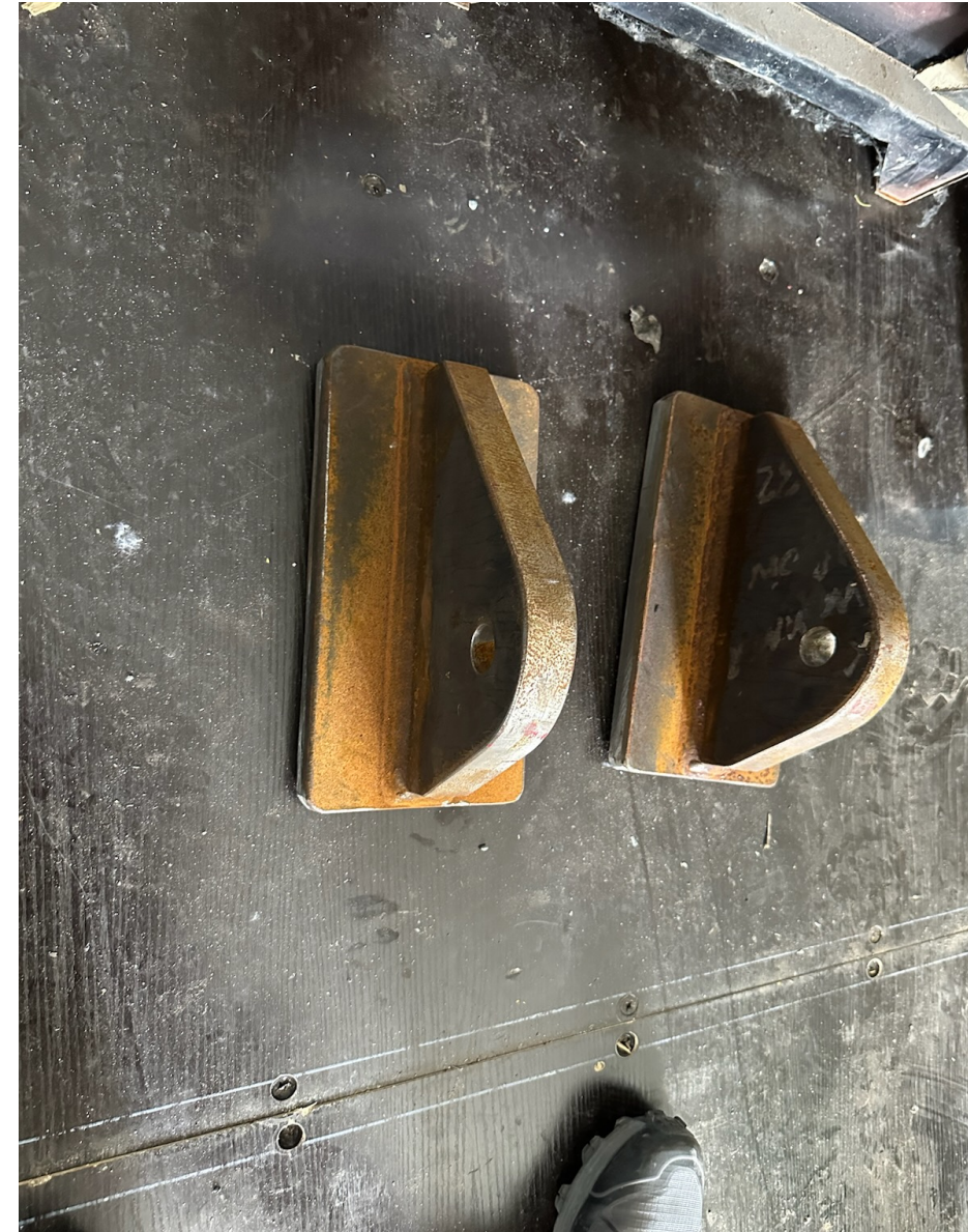
12" x 6" attachment plates for stiff-leg attachment to concrete
