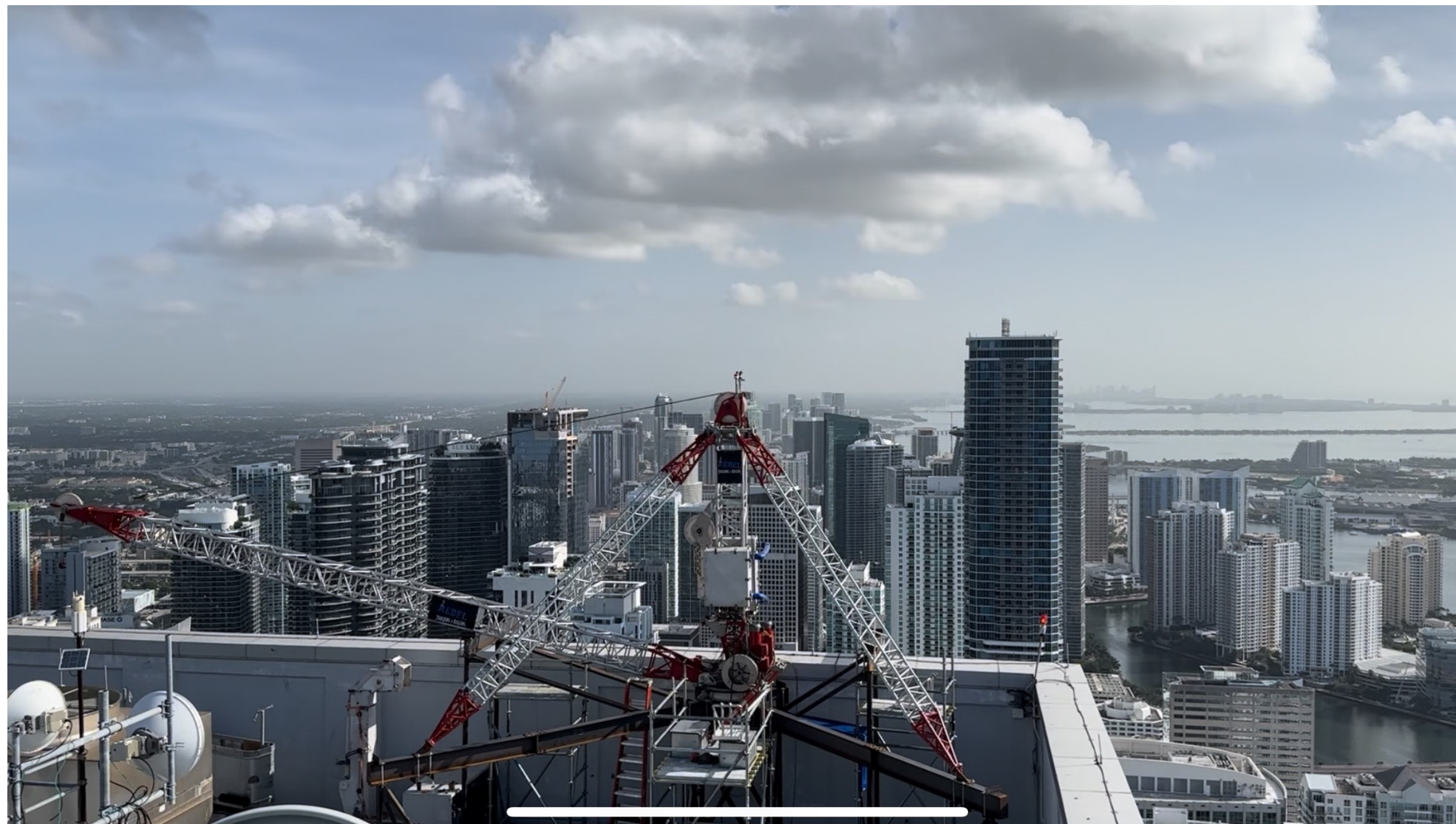
LSC on support beams 820' above sidewalk
