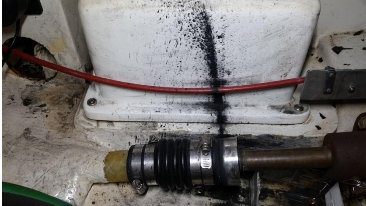
Shaft Seal/Sling Mark Finding
