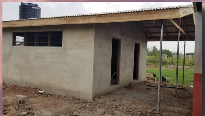
New School Building
