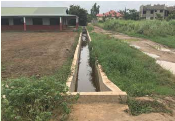
NEW Drainage Gutter at the School
