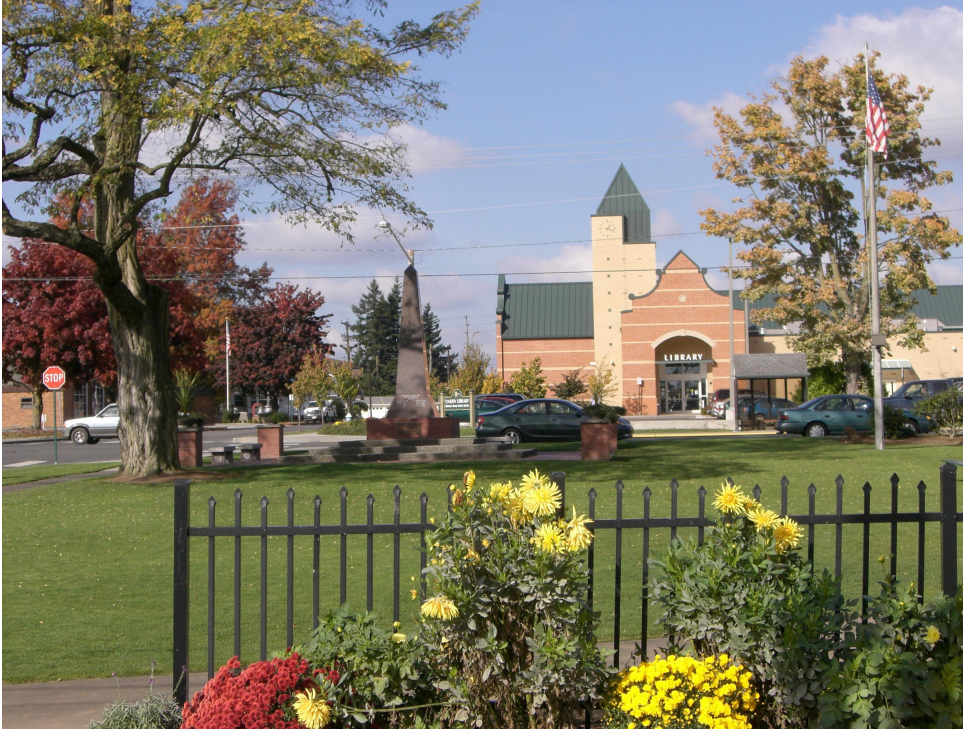
Lynden, WA Public Library. Set one block off Lynden’s mainstreet with a green community commons, memorial, and public transportation stop is an example of an honorific civic building that references community history. (Received a +5 VDS survey result)
