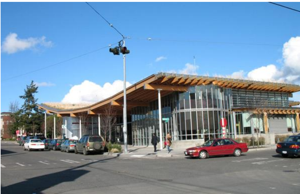
Ballard Library and Neighborhood Service Center, Seattle WA. Set one block off a historic neighborhood main street this civic building has a library, community meeting room for 75, local court and police services, and civic administrative services.
