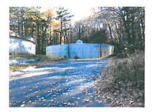
The Reeves Hill Water Storage Tank No. 2 is a prestressed concrete tank constructed in 1958. This tank was cleaned in 2002. The tank was inspected in 2006 and was considered to be in very good condition. The Wayland Water Department is planning to power wash the tank in the summer of 2008.
