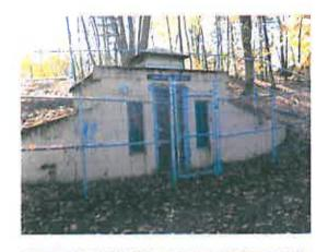
A new building was constructed near the Well No. 1 building for chemical storage in 1999. All of the chemicals for Well No. 2 are stored here, along with some of the chemicals for Well No. 1. Chemical injection occurs in a manhole outside of the building.
