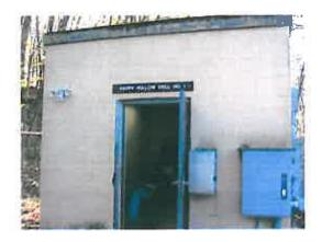
Happy Hollow Well No. 2 was originally installed in 1951 in a concrete building with a concrete slab roof. The pump motor was rebuilt in 2006, but it is unknown if the pump has been replaced. No repairs have been made to the roof or building since construction. The 2007 well inspection report claims that the well and pump appear to be in good condition.
