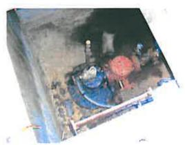
Well No. 3 was installed in 1955 and is located in a concrete building with a concrete slab roof installed in 1998. The pump and pump motor were replaced in 1993. The well was redeveloped in 1998. The 2007 well inspection report recommends the pump be pulled and inspected. Chemical storage and injection was added to the building in 1999.
