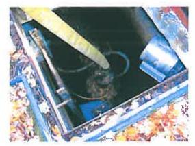
Well No. 2 was installed in 1944. The current pump was installed in 1993 and the pump motor was replaced in 2003. The pump and motor are located in the original concrete vault. The well was inspected in 2007 and found to be in good condition. Well No. 2 is currently offline due to high iron and manganese levels.
