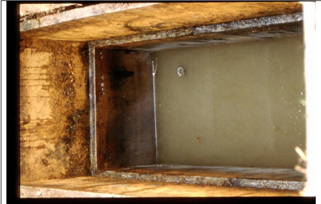
Figure 6.7 Water-Filled Concrete Vault at CEN
