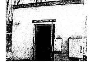
Happy Hollow Well No. 2 was originally installed in 1951 in a concrete building with a concrete slab roof. The pump motor was rebuilt in 2006, but it is unknown if the pump has been replaced. No repairs have been made to the roof or building since construction. The 2007 well inspection report claims that the well and pump appear to be in good condition.
