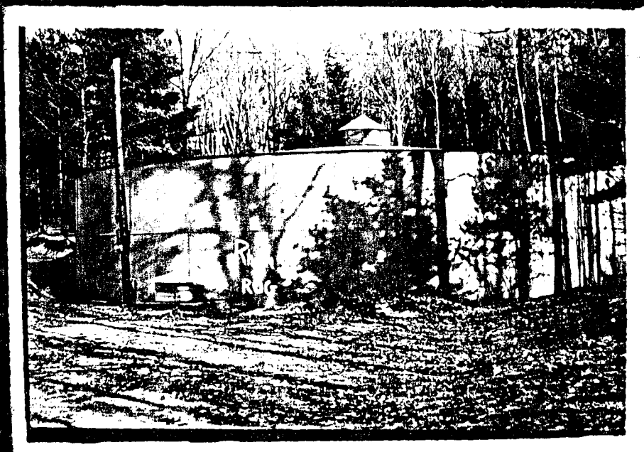
This was the first of the two standpipes build on Reeves Hill in 1927. It has a capacity of 500,000 gal. Its elevation is 357 ft. above sea level and is made out of steel frame and panel.
