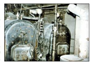
the back driveway) to the boilers. This was hard, time-consuming labor. Manville Kendrick recalled that an automatic stoker – a device that supplied fuel to the boilers by mechanical means – was installed in the 1920s.
