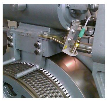
Figure 23: Installed ETSD Tape & Sensor
