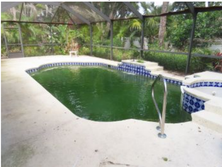
Exterior Areas Swimming Pool & Enclosure
