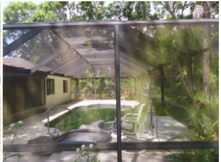
Exterior Areas Swimming Pool & Enclosure
