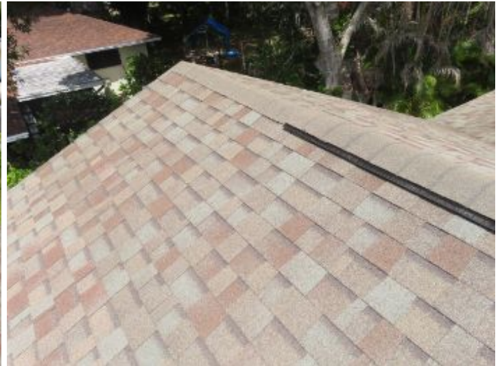
Exterior Areas Roof
