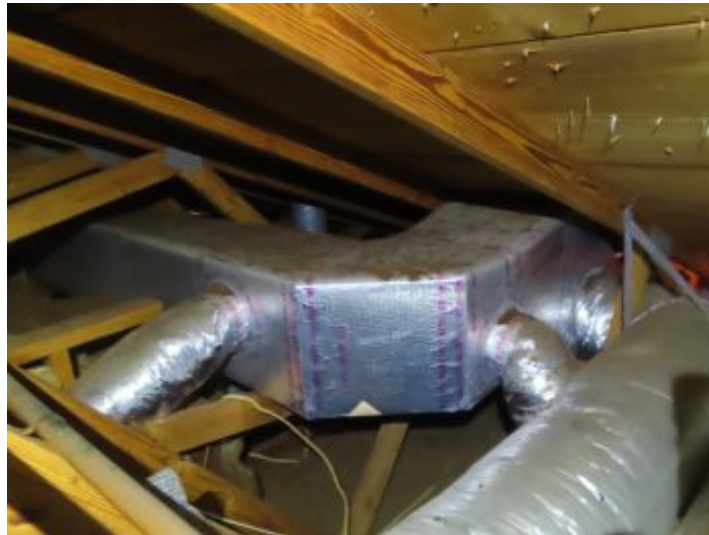
Garage,Attic, Structural & Foundation Attic
