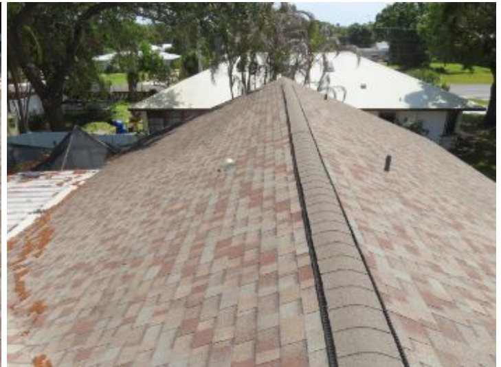
Exterior Areas Roof
