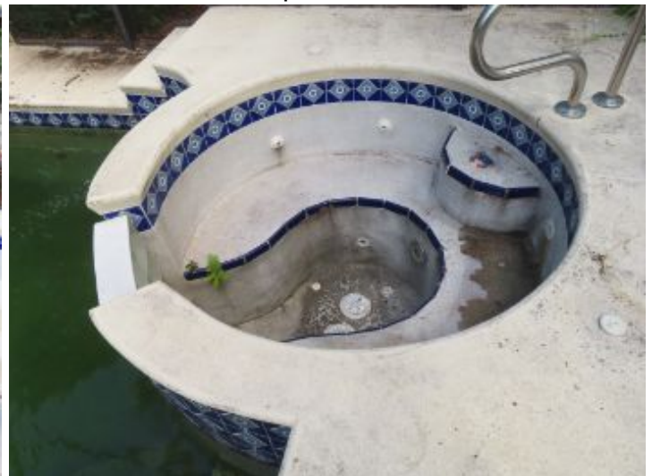
Exterior Areas Swimming Pool & Enclosure
