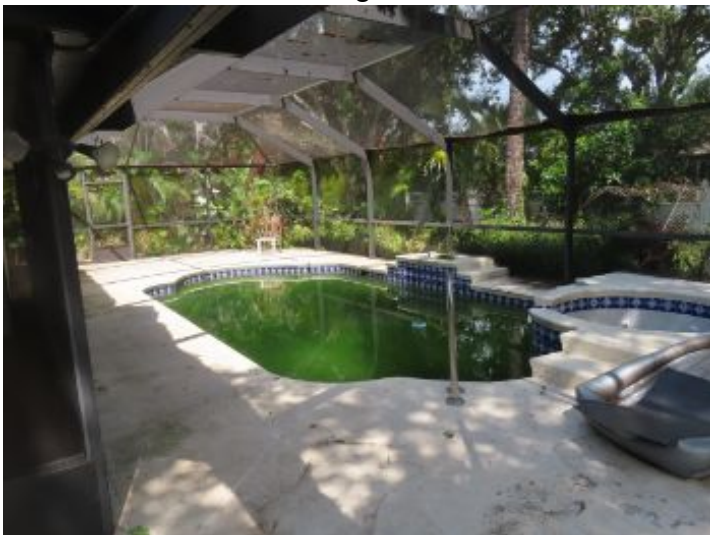
Exterior Areas Swimming Pool & Enclosure
