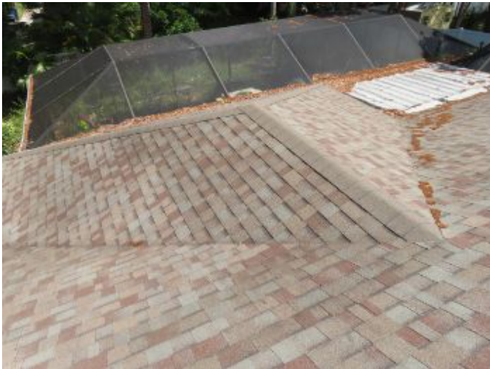
Exterior Areas Roof
