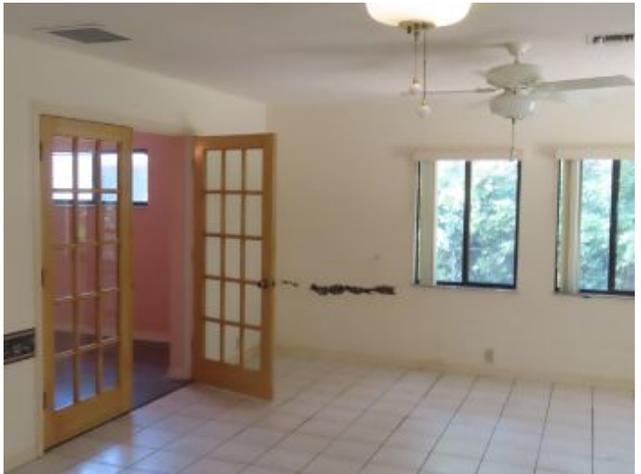
Interior Features Interior Areas
