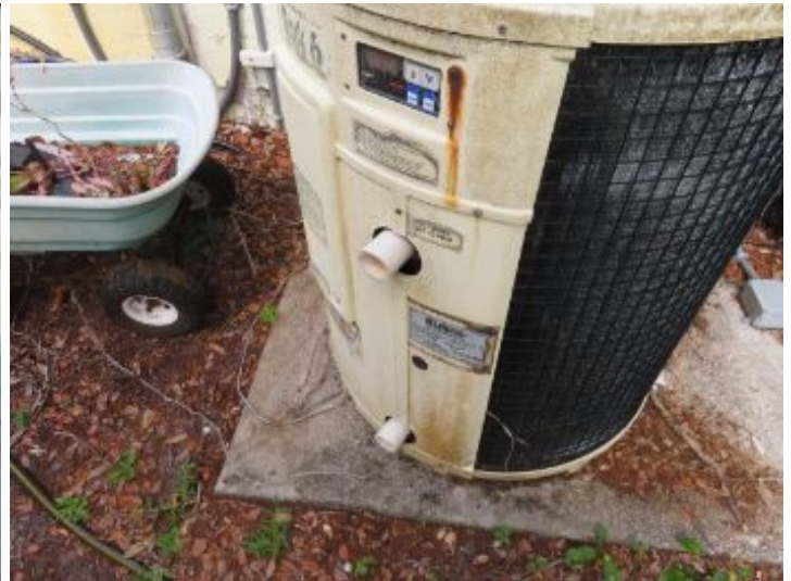
Exterior Areas Swimming Pool & Enclosure
