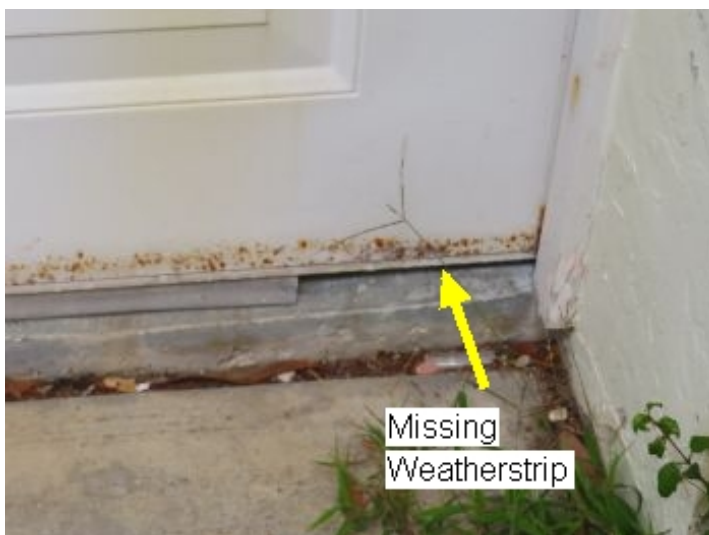
Rust on garage door skin - Missing part of bottom OHGD is missing weather stripping - Light shining through
