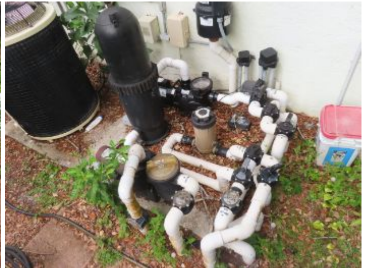
Exterior Areas Swimming Pool & Enclosure
