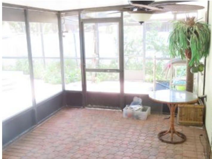
Exterior Areas Covered Porch
