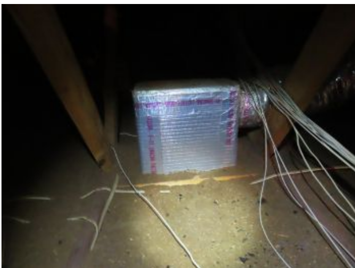
Garage,Attic, Structural & Foundation Attic
