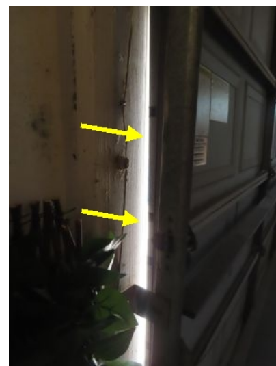
Rust on garage door skin - Missing part of bottom OHGD is missing weather stripping - Light shining through
