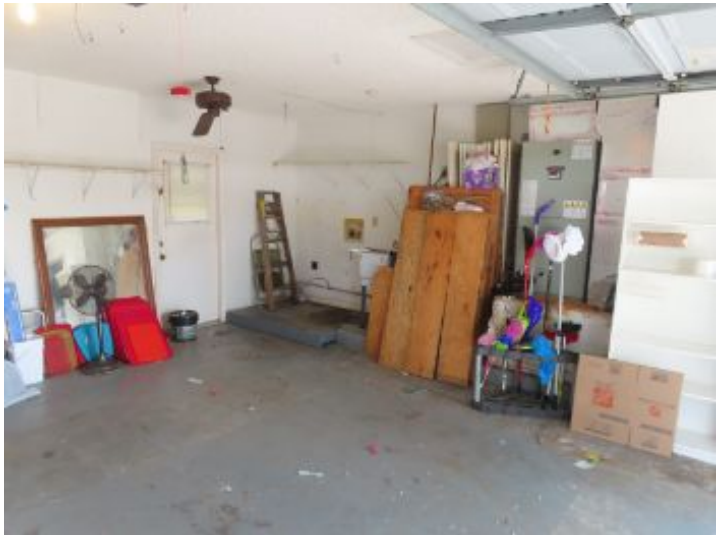
Garage,Attic, Structural & Foundation Garage
