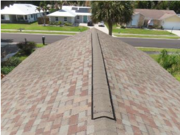
Exterior Areas Roof
