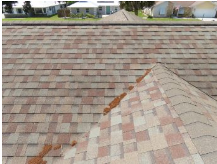
Exterior Areas Roof
