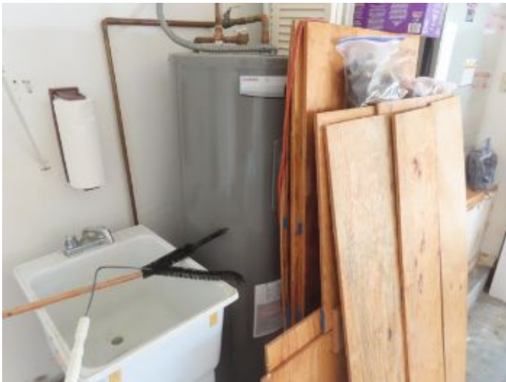
Garage,Attic, Structural & Foundation Garage
