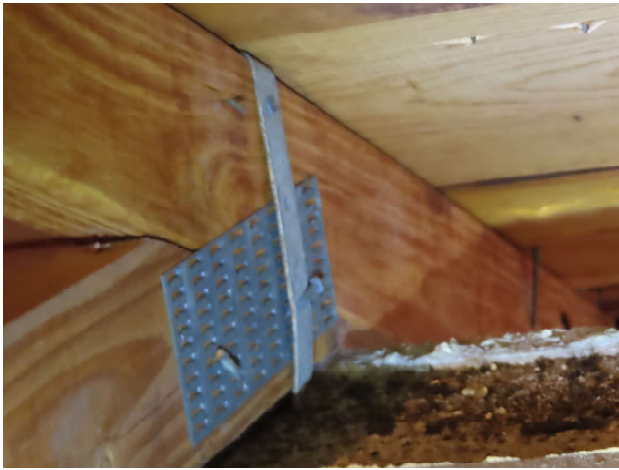
Roof to wall attachment - Single wrap
