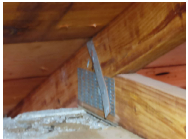
Roof to wall attachment - Single wrap
