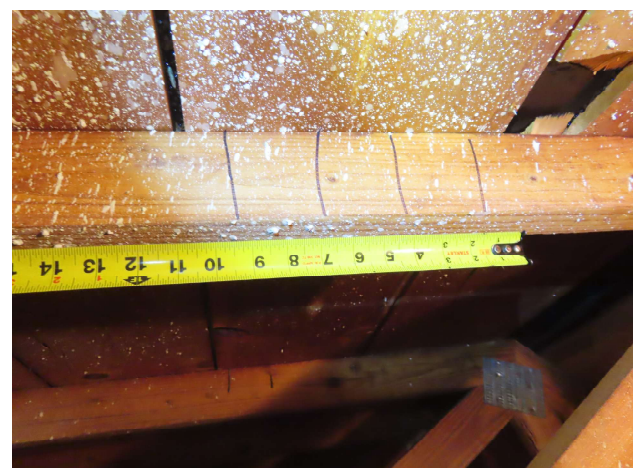
Roof deck nail spacing - 4 nails per bd
