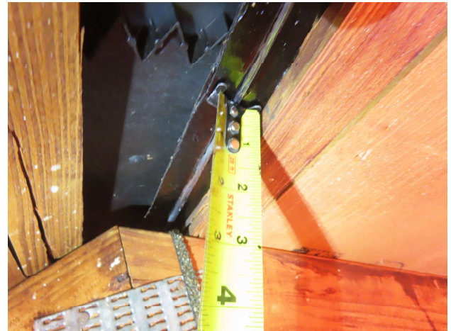
Roof deck - 3/4" planks
