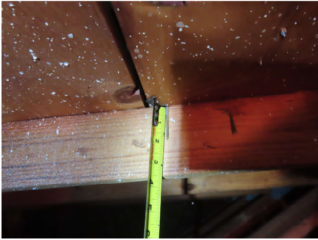
Roof deck attachment - 8d nails
