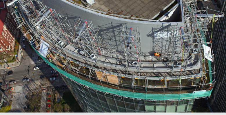
The netting attached to the suspended deck prevents spillage for the One Wall project.
