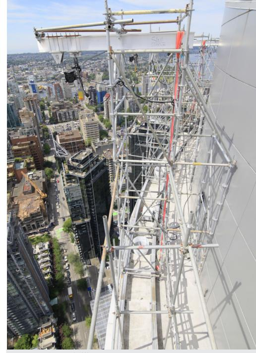
The custom platform is a 4'x400' long, multi-point suspended work platform that weighs 18,368 lbs.
