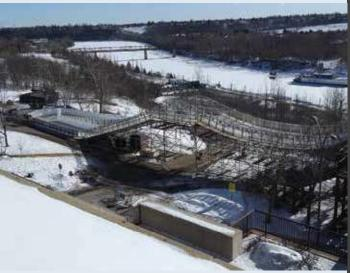
As well as the track itself, Matakana Scaffolding also constructed camera towers and lighting, PA, and viewing screen support scaffolds. It is hoped that the Crashed Ice Race will be held again in Edmonton sometime in the next 5 years.
