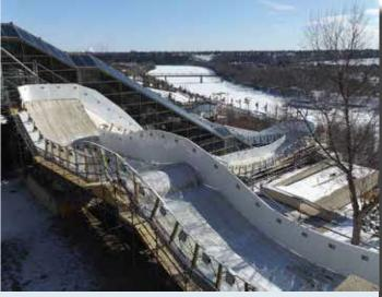
The track build had to revolve around the normal daily activities of the Convention Centre and had to bridge over access roads and streets. An ice surface was created on the track and 36,000 liters of coolant piped through the refrigeration system.
