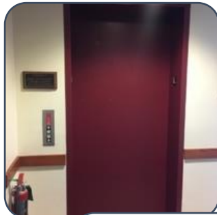
1996 Elevator installed in the church.
