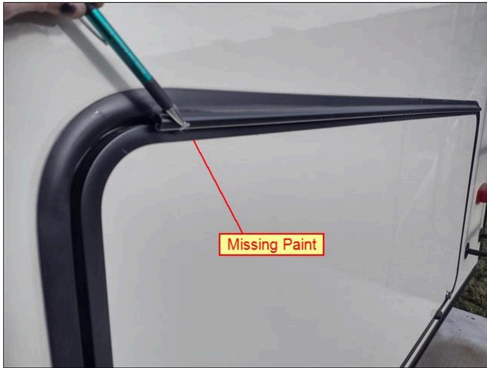
Missing Paint on Rear Cap Access Door Hinge.
