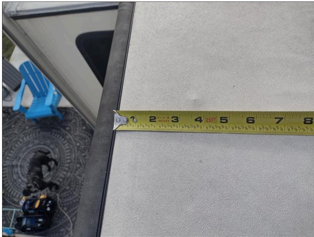
First Location 4" from edge of Curbside directly above entry door.
