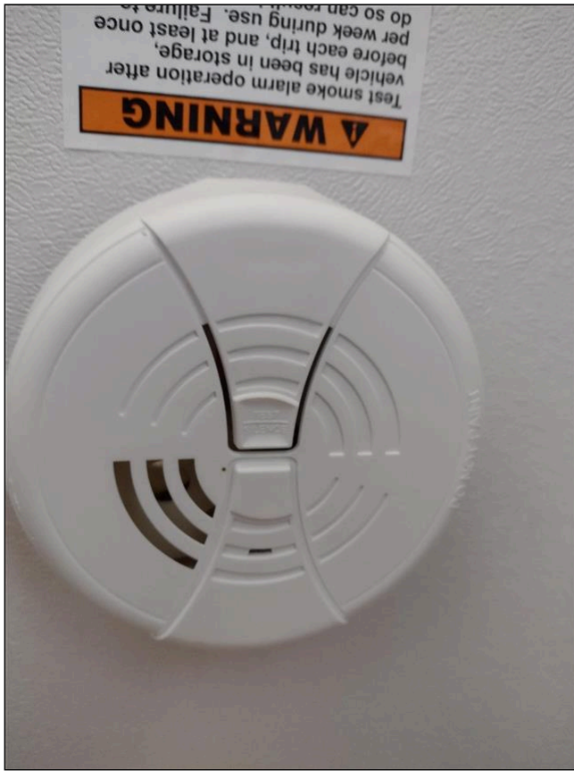
Hallway Fire Detector Front
