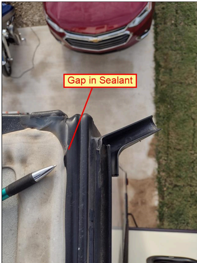
Streetside Rear Cap Seal - Gap in Sealant
