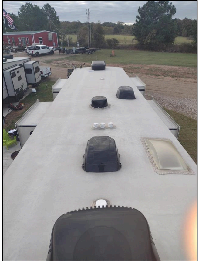
Roof Overview - Front to Back
