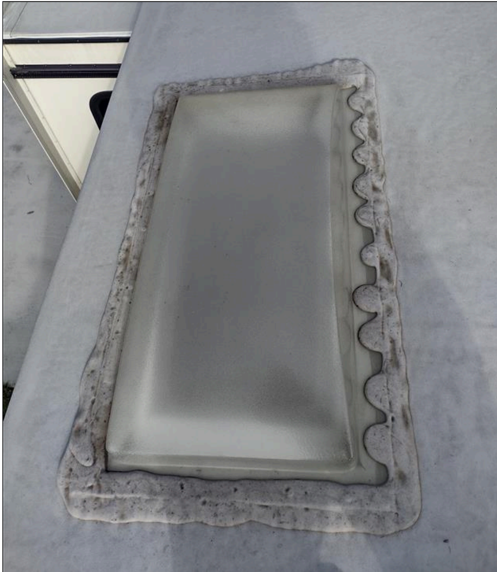
Shower Skylight - Streetside
