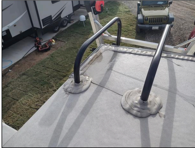
Curbside Rear Cap Seal - Standing Water
