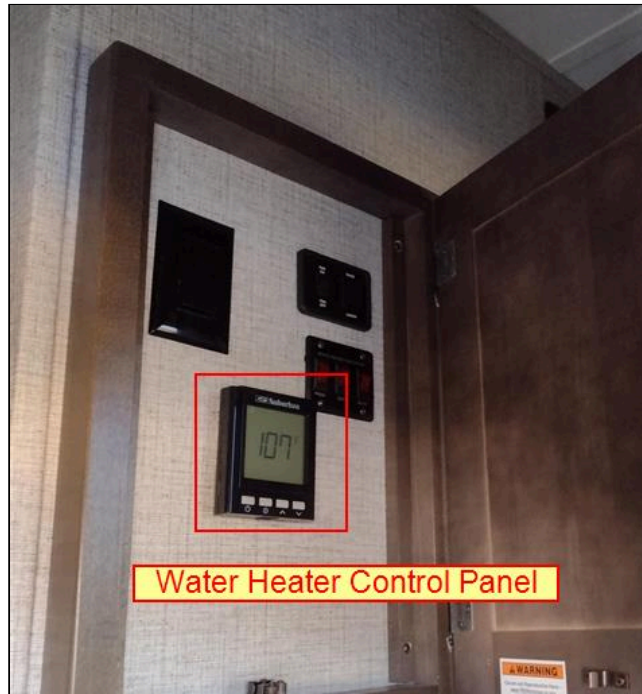
Water Heater Controls
