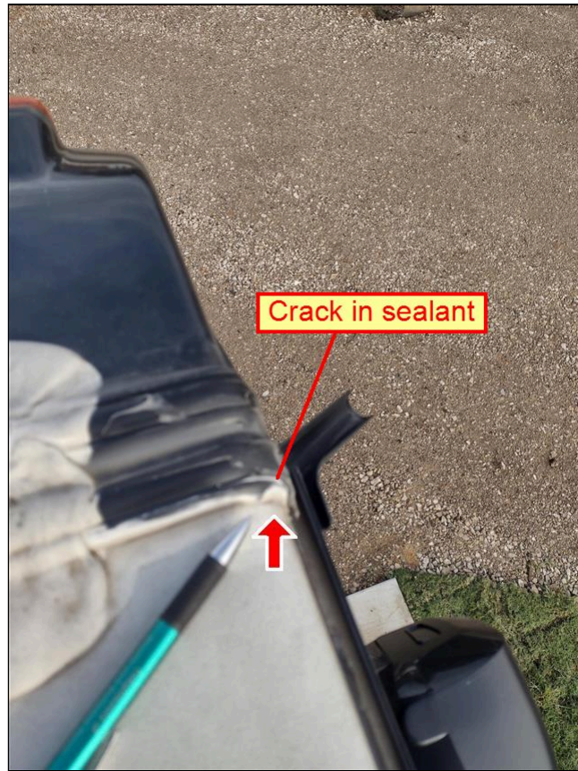
Front Curbside Cap Joint Corner
