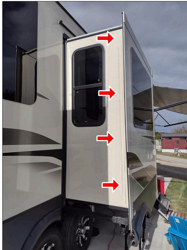
Curbside Center Slideout - Black Residue
