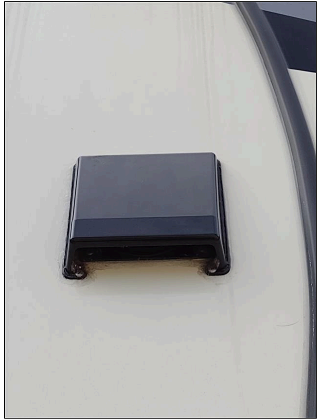
Dryer Vent Condition
