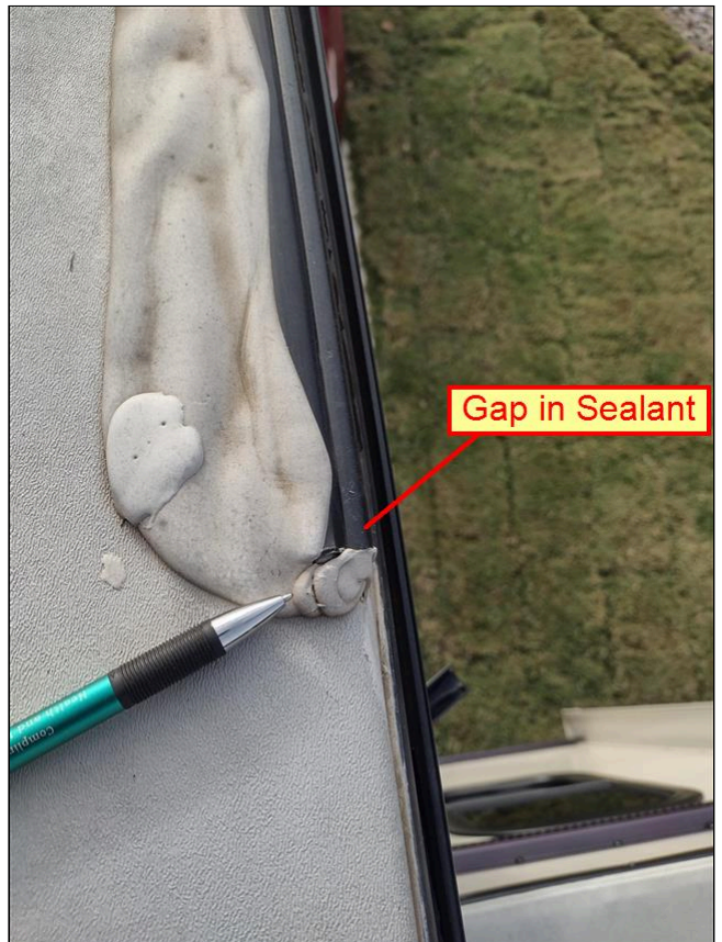
Streetside Rear Cap Seal - Gap in Sealant
