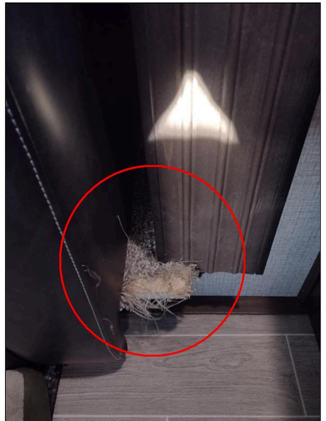
Carpet Damage Right Side of Sofa
