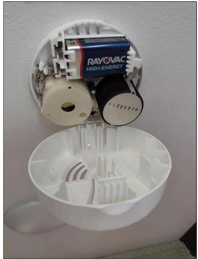
Hallway Fire Detector Inside
