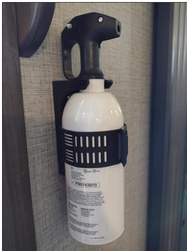
5 B:C Fire Extinguisher
