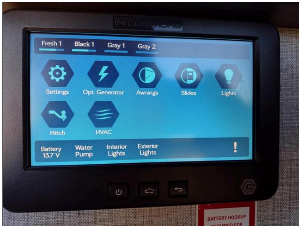
Battery / Waste / Water Monitor Panel
