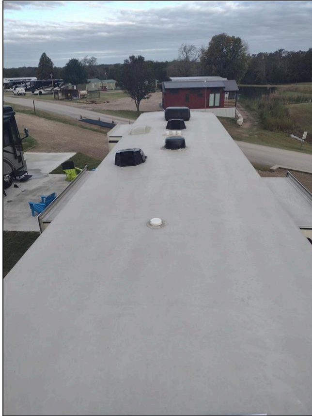
Roof Overview - Back to Front
