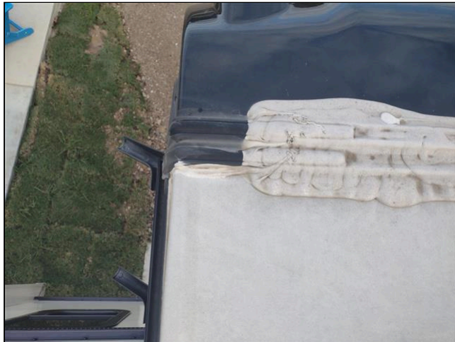
Streetside Front Cap Joint Corner
