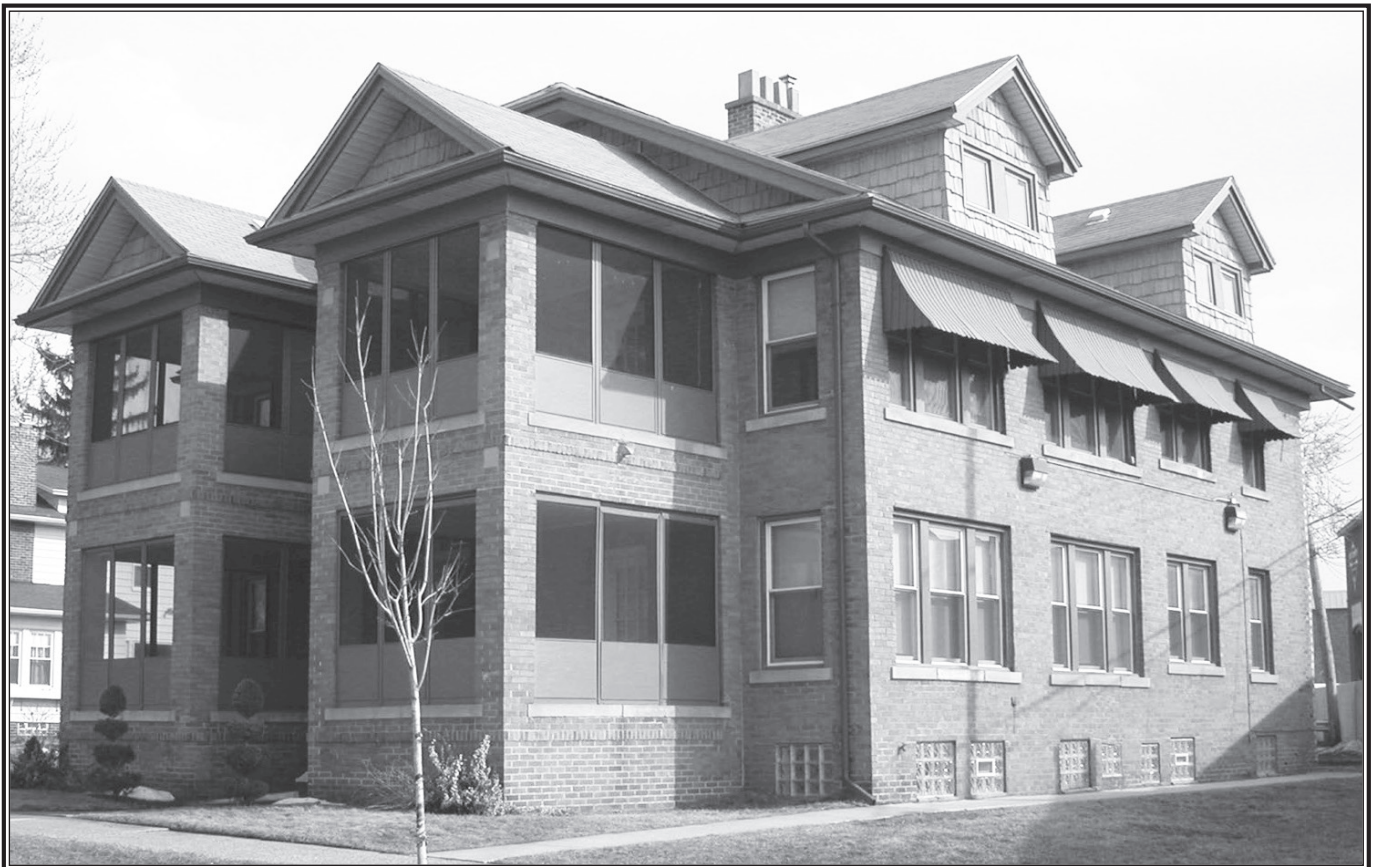
The building has two kinds of common brick: yellow raked brick shown on the left, and common red brick on the right.
