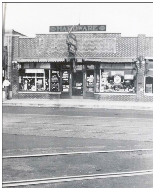
View of the store from Catalpa, with streetcar tracks in foreground, c. 1935.
