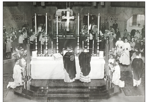
Priests gather around the 18½-ton main altar, carved from a single block of Carrara marble from Italy. Note that presiders now stand on the opposite side of the altar than in this photograph.
