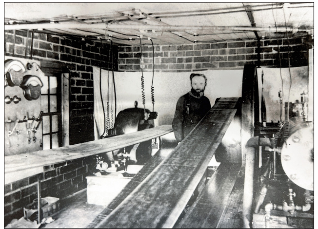
Hilzinger in the power plant he built in 1901 after the milk station closed. Gasoline engines generated the electricity.
