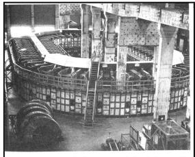
54. Oak Ridge Alpha I calutron racetrack for electromagnetic separation of U235. Silver-wound magnets protrude like ribs spaced by semicircular mass-spectrometer tanks. Spare tanks in left foreground.
