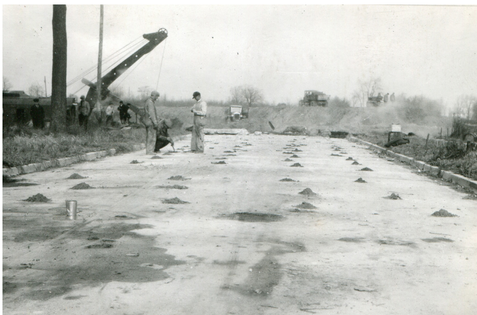
Placing dynamite ready for blowing pavement to grade Glenview Avenue to new level of Webster Road, circa 1930. Photo courtesy of Royal Oak Historical Museum
