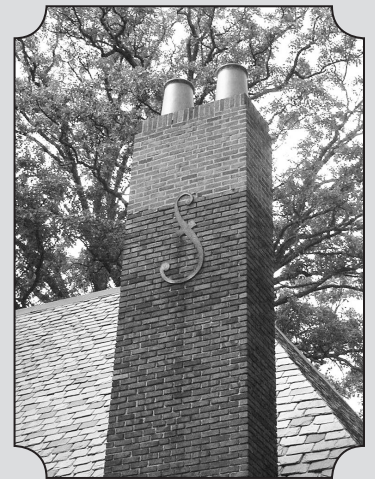
The "S" for "Starr" on the chimney.
