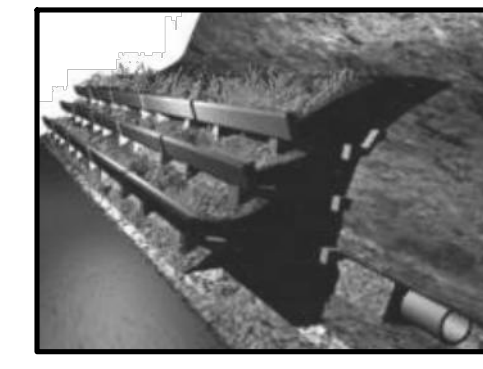
PHOTO OF WALL JUST AFTER INSTALLATION AND PLANTING
