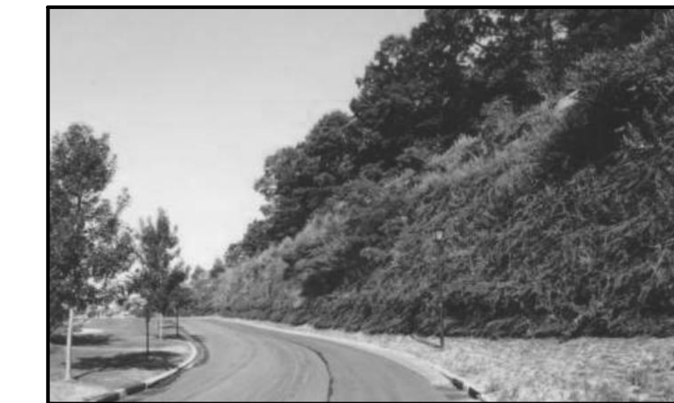
PHOTO OF WALL BEHIND FULL GROWTH VEGETATION
