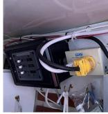
**General Condition of Wiring and Fixtures:** Would benefit from installation of an ELCI. (see 4)
