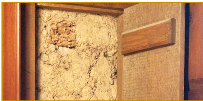
Original adobe construction beneath wooden walls. It's possible this adobe was from the original Hollingshead homestead.†
