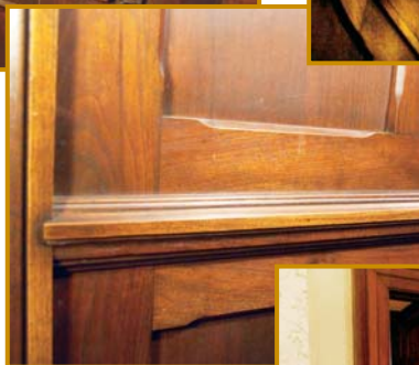
There are many examples of the original panelling, doors and windows throughout the house. †
