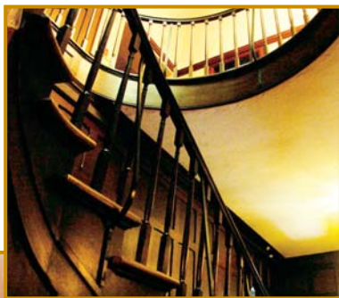
Crookshank's stair rails & posts. †
