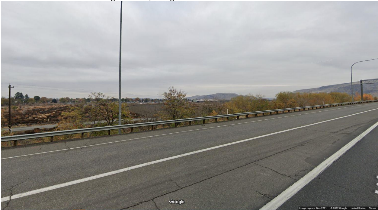
Photo 5: Intersection-82- existing condition, facing west
