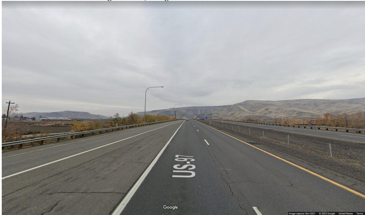
Photo 6: Intersection-82- existing condition, facing north
