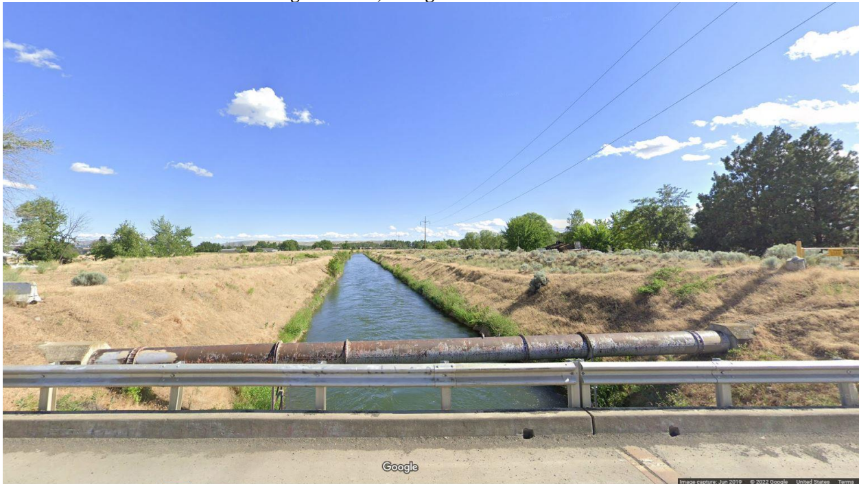
Photo 11: Eastmost terminus- existing condition, facing south
