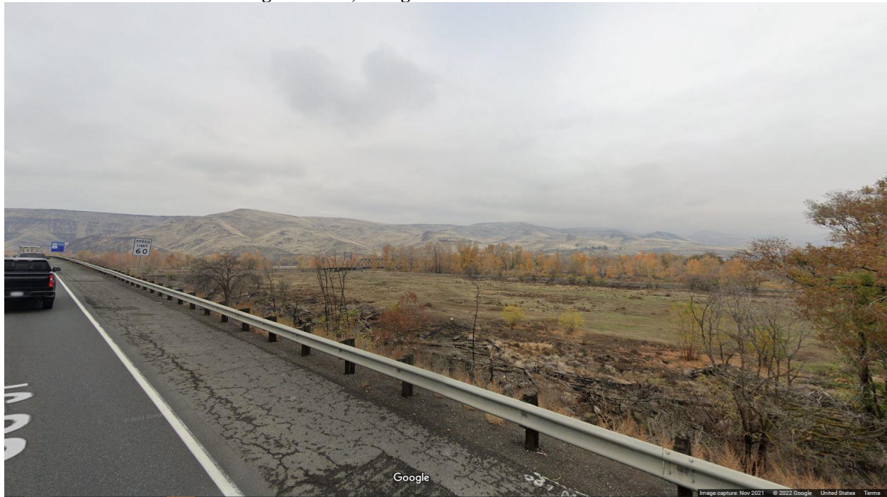
Photo 4: Intersection-82- existing condition, facing northeast
