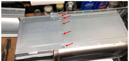
D. Drill and screw the extension rear wall to the dedicated oven by drilling 5 holes through the extension box rear wall and dedicated oven rear wall and attach with 5 screws (red arrows below).
