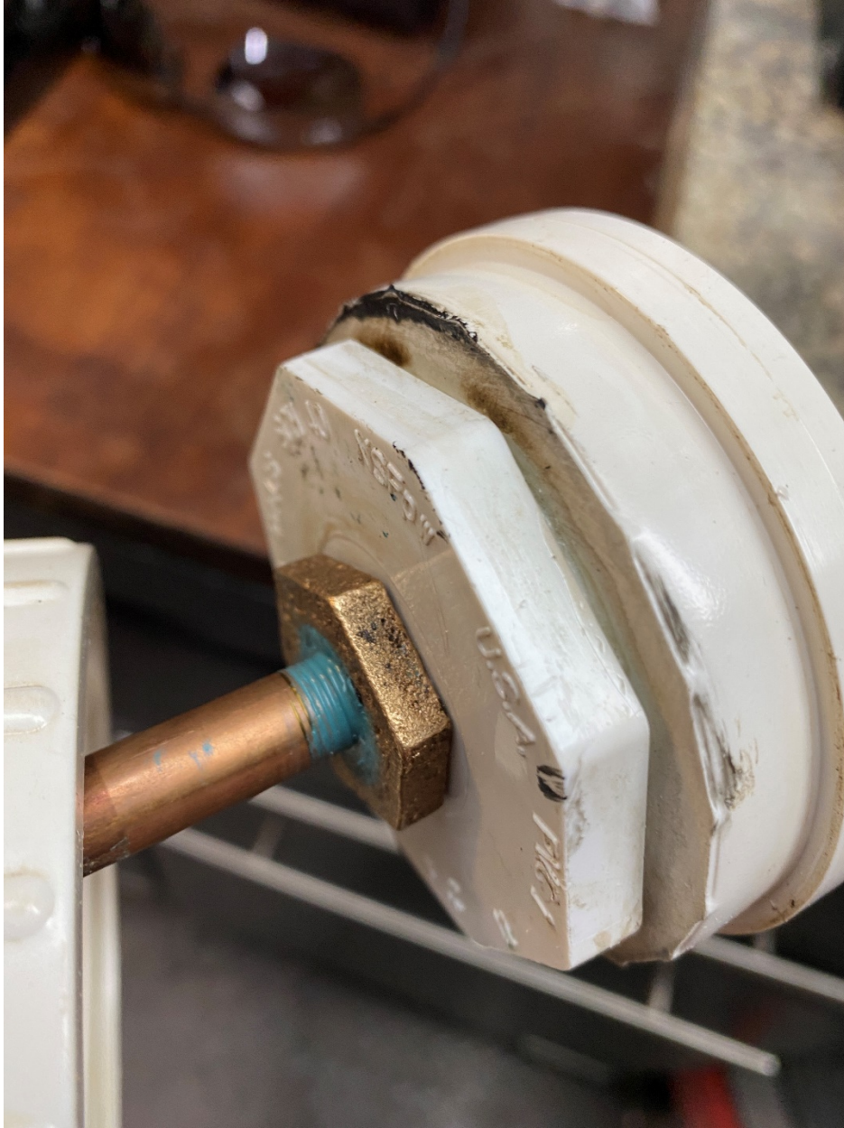
Another view of cut down PVC adaptor glued into Union. This is the top of the Union where the grease gun is now attached with a brass nipple to the brass adaptor. This is much better than the original hose.
