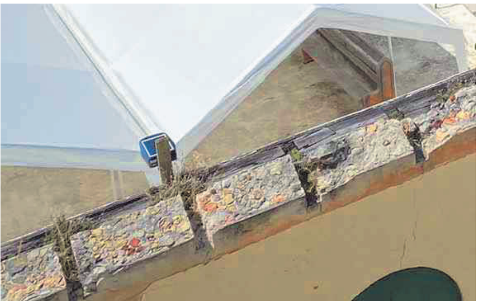
EXISTING RAFTER/TRUSS SLOTS
