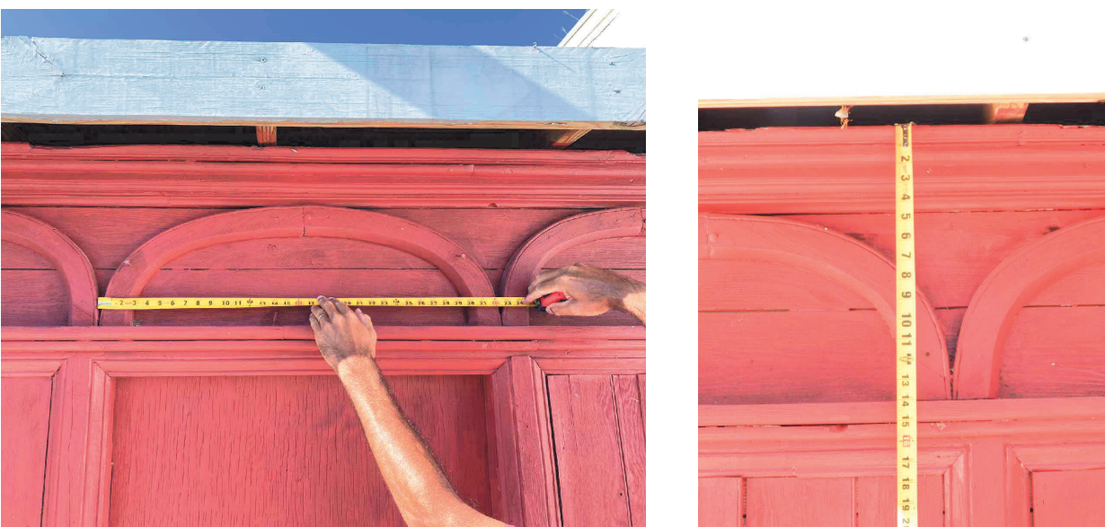
EXISTING VESTRY TRIM PHOTOS
