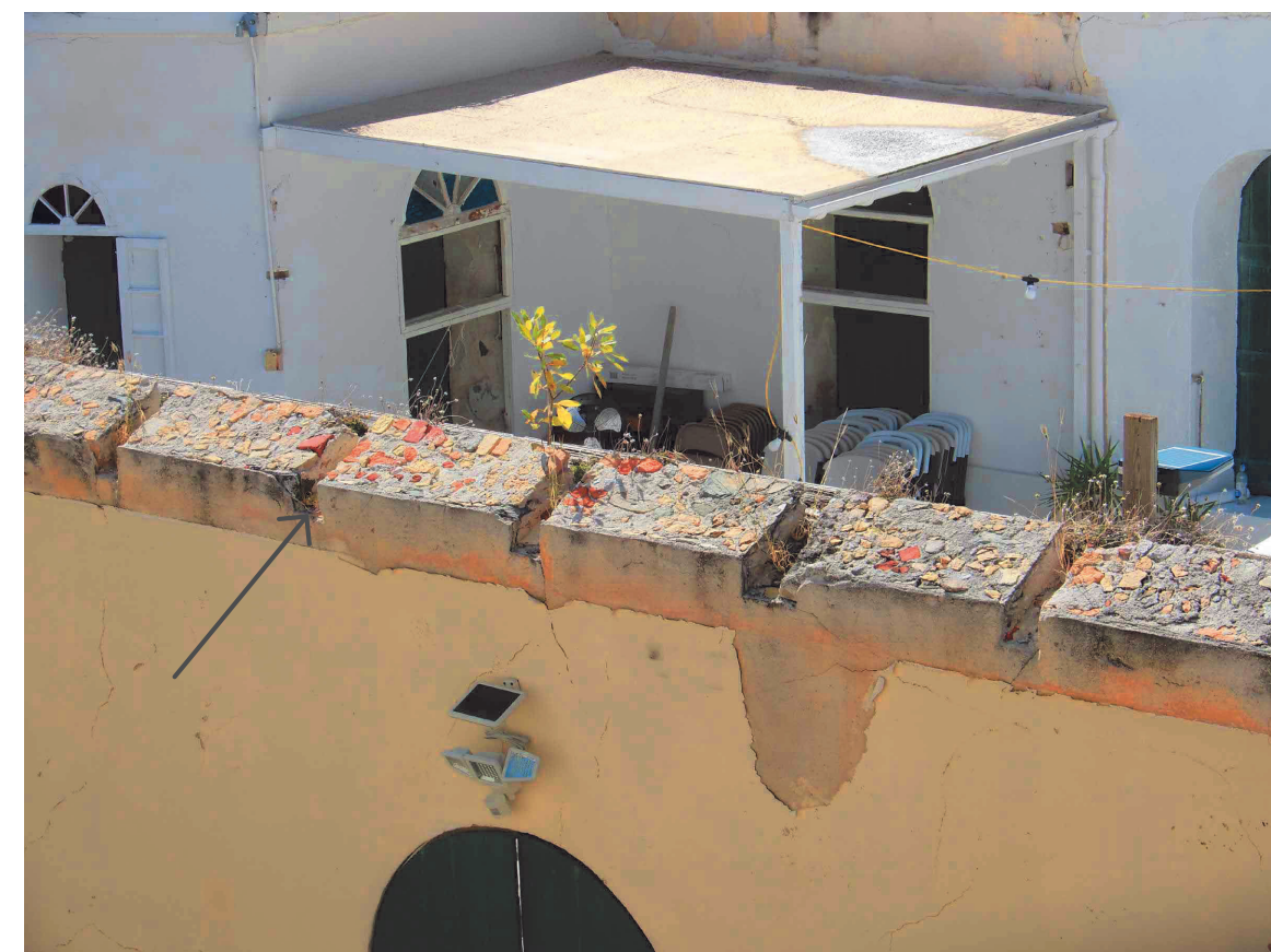
EXISTING RAFTER/TRUSS SLOTS
