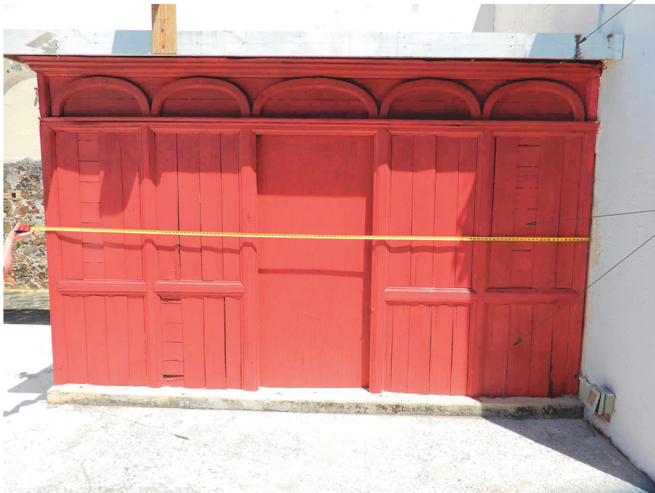
VESTRY EXISTING NORTH ELEVATION PHOTO
