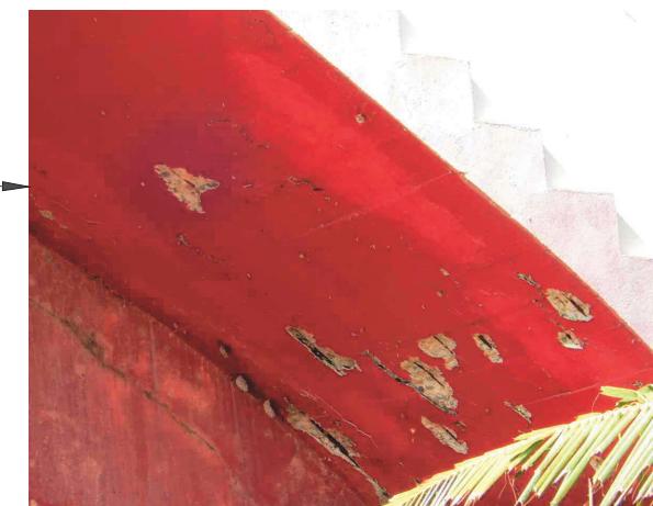
EXPOSED REBAR @ UNDERSIDE OF STAIR
