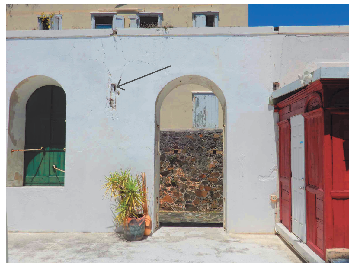
EXISTING PRIMARY TRUSS EMBEDMENTS
