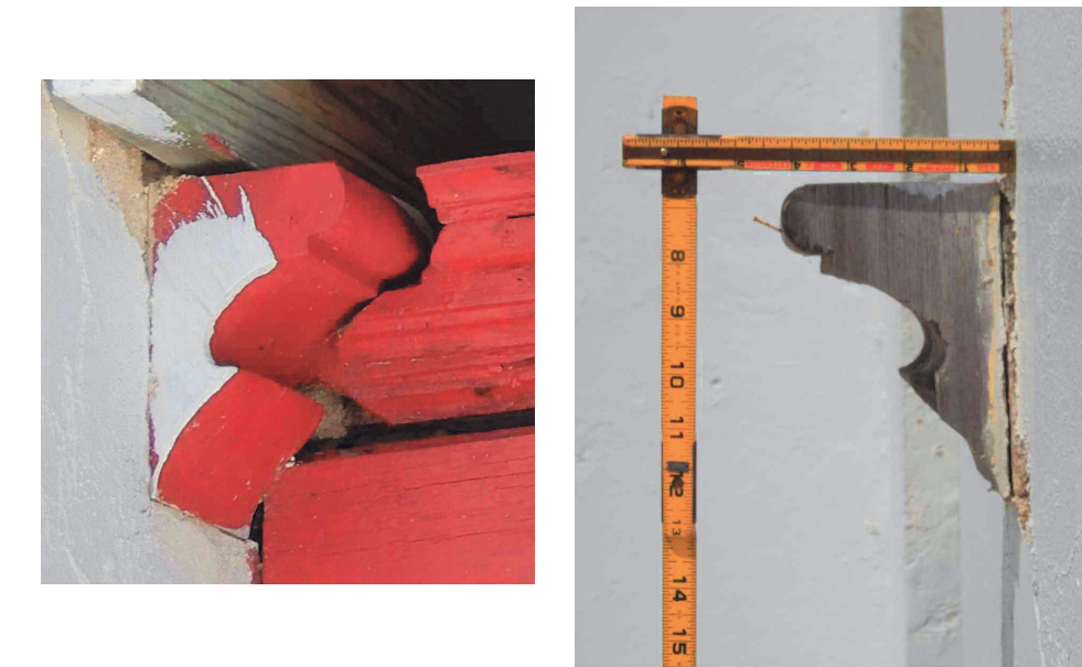
PHOTO OF EXISTING TRUSS BASE
