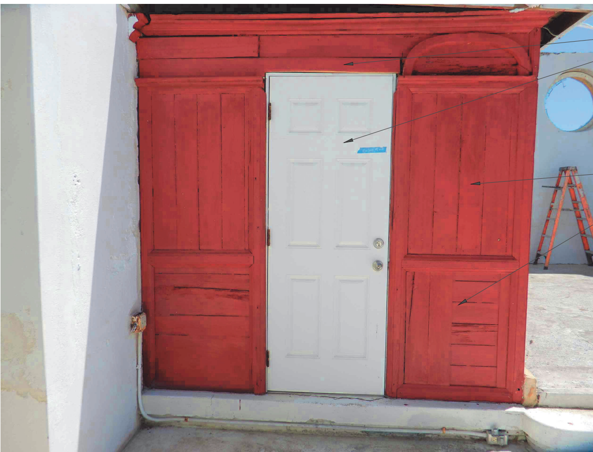
VESTRY EXISTING EAST ELEVATION PHOTO
