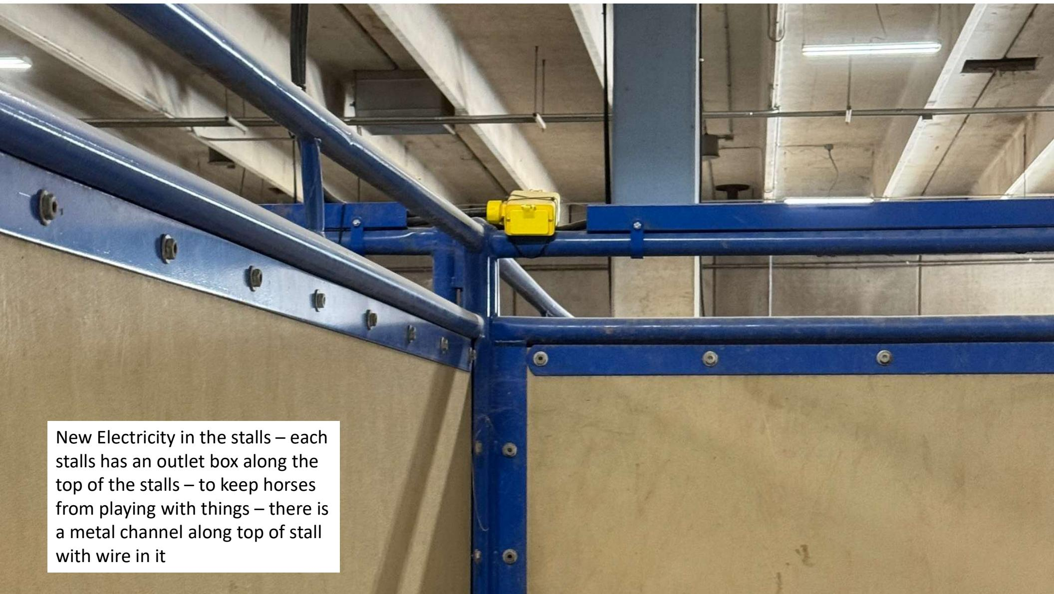
New Electricity in the stalls – each stall has an outlet box along the top of the stalls – to keep horses from playing with things – there is a metal channel along top of stall with wire in it
