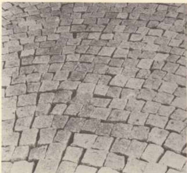
Cobblestone street completed by Winston-Salem Paving Co.
