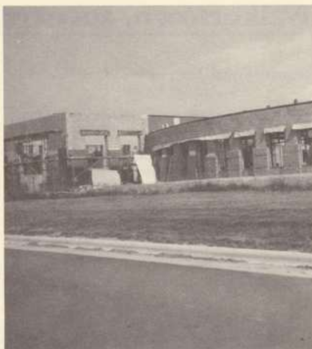
Library under construction
