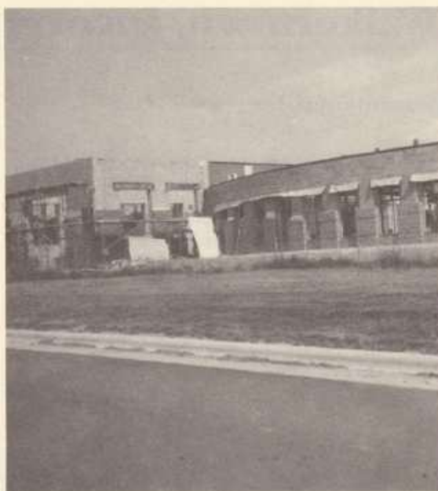
Library under construction
