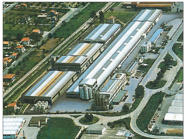
Alfagomma Rubber Industrial Hose Manufacturing facility – Teramo, Italy
