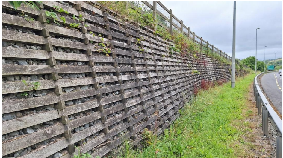
Figure 7: Crib retaining wall beside a national roadway
