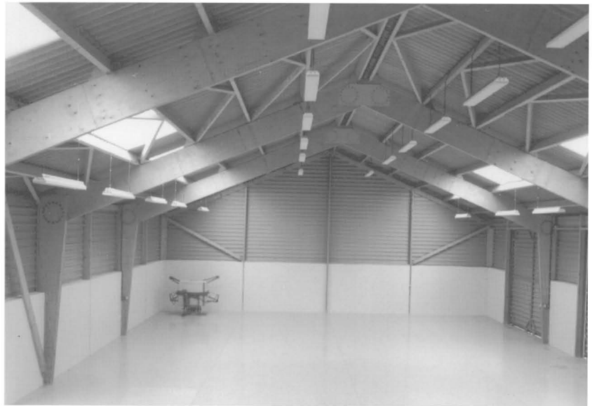
Figure 5 LVL frame communal workshop, Sixt-Sur-Aff, France. Span 18 m.
