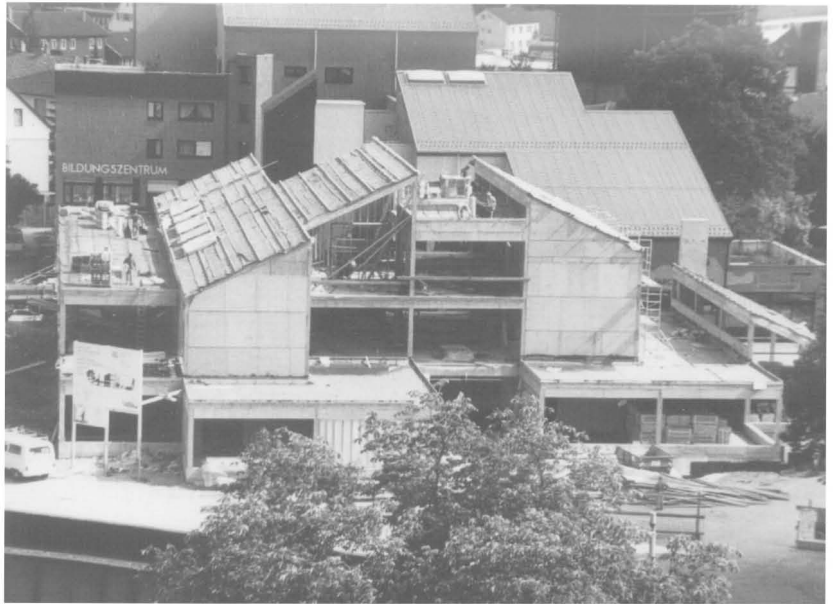
Figure 4 Albstadt Centre for Technology and Economics, Germany: earthquake resistant shear walls made of cross-veneered LVL panels.
